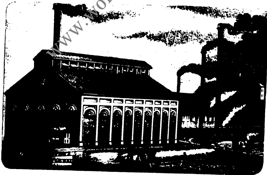
OPEN HEARTH FURNACE AND BLOOMING-MILL, PENNSYLVANIA STEEL-WORKS.
