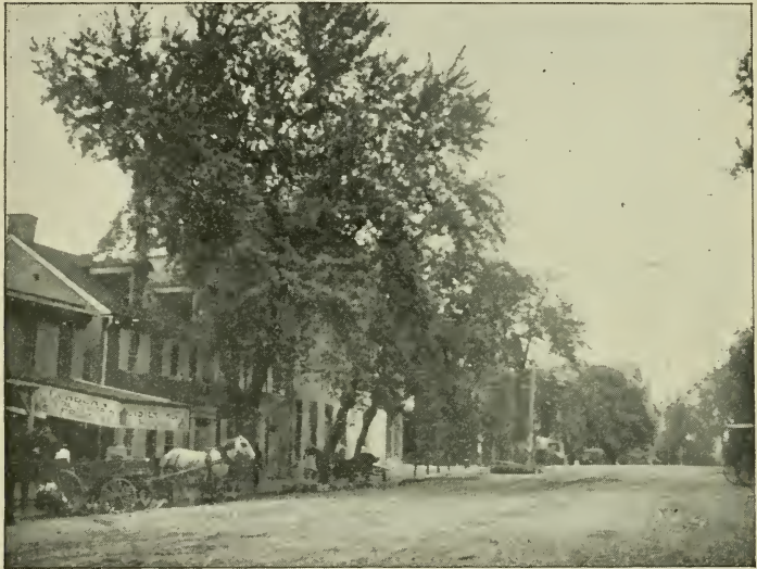
CENTRAL SQUARE, LEBANON, PA.
