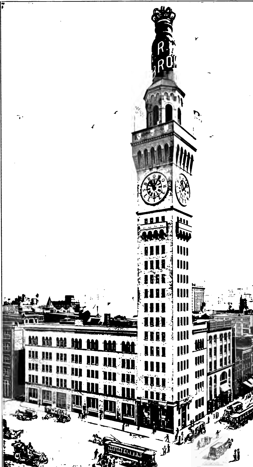
BROMO-SELTZER TOWER. Total height of tower, 357 feet. The Bottle on top, a fac-simile of the regular ten-cent Bromo-Seltzer bottle, but about 10,000,000 times larger, is 51 feet high, 20 1/2 feet in diameter, weighs 17 tons, and revolves at the rate of 107 feet per minute. There are 506 electric lights in bottle and crown surmounting it, which can be seen at a distance of 20 miles. The Bromo-Seltzer clock is the largest four-dial gravity clock in the world. The dial is 24 feet in diameter. The minute hand is 12 feet 7 inches long, and weighs 175 pounds. The hour hand is 9 feet 8 inches long and weighs 145 pounds. The pendulum is 15 feet long and weighs 475 pounds. The clock is automatically wound by an electric motor every six hours.
