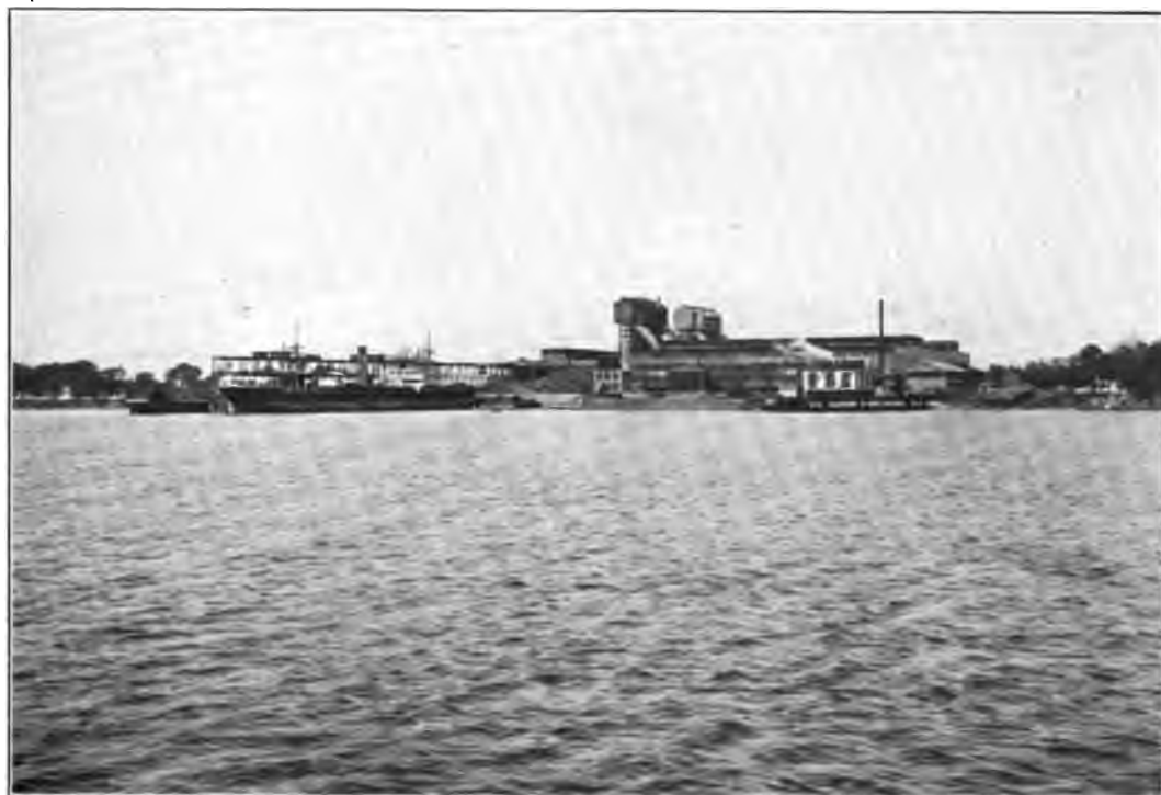
DAVISON CHEMICAL COMPANY , Curtis Bay plant.
