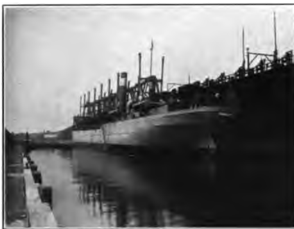
COAL PIER, CURTIS BAY.
