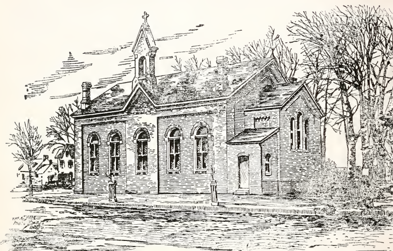
EMMANUEL P. E. CHURCH, CHESTERTOWN, MD., BEFORE IMPROVEMENTS ADDED.
