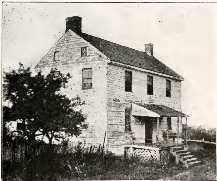
"FISH HALL," THE FIRST HOUSE BUILT IN BETTERTON, IN 1698, AND OWNED BY EDW. CREW.
