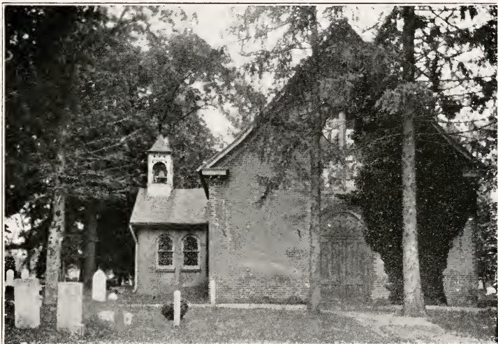
ST. PAUL'S, BUILT IN 1713, IS THE OLDEST BUILDING IN THE STATE USED CONTINUOUSLY AS A PLACE OF WORSHIP. THE "VESTRY HOUSE," BUILT IN 1776, IS AT THE LEFT.
