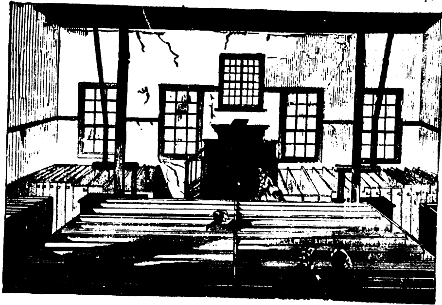
INTERIOR VIEW OF OLD DERRY CHURCH.
