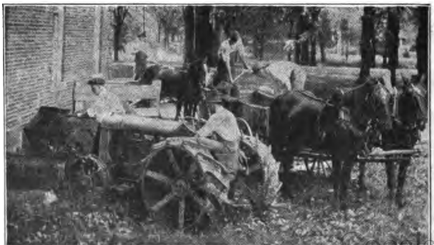
Students laying concrete base in Science Hall, Blackburn College, Carlinville, Illinois.
