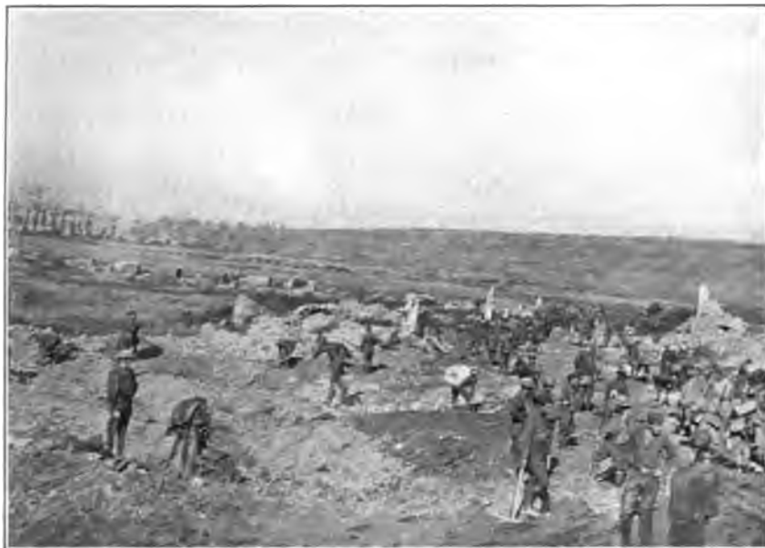
104TH ENGINEERS WORKING ON ROAD THROUGH SAMOGNEUX, OCT. 18, 1918.
