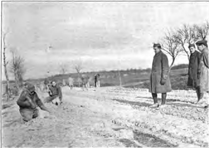
104TH ENGINEERS REPAIRING FRENCH ROADS IN THE 11TH AREA AFTER THE ARMISTICE.
