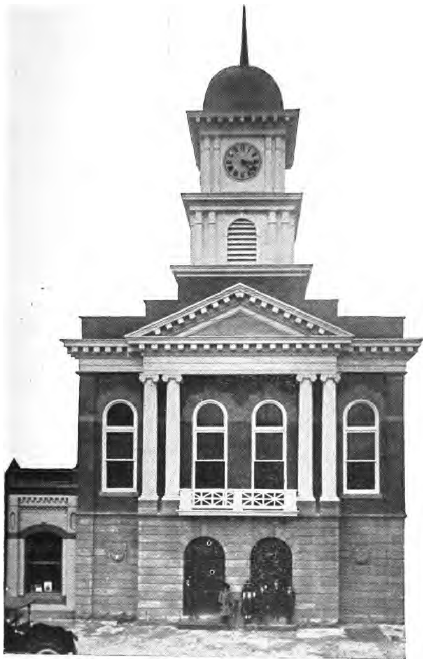
The above is a likeness of the front of the Snyder County Court House, as remodeled during the year 1916. The original Court House was built in the years following 1855, when Snyder County was formed. This was remodelled and enlarged in 1867 at a cost of over $11,000.
