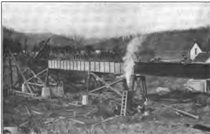
Dent's Run Bridge.
