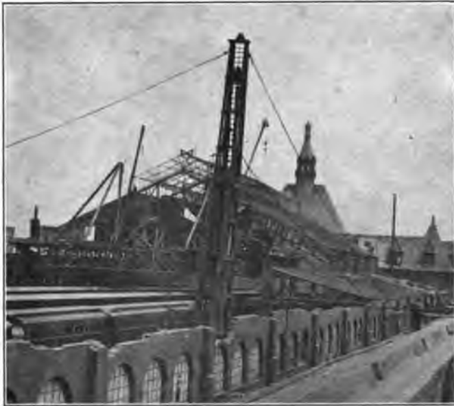
Dismantling of Train Shed Nearing Completion.
