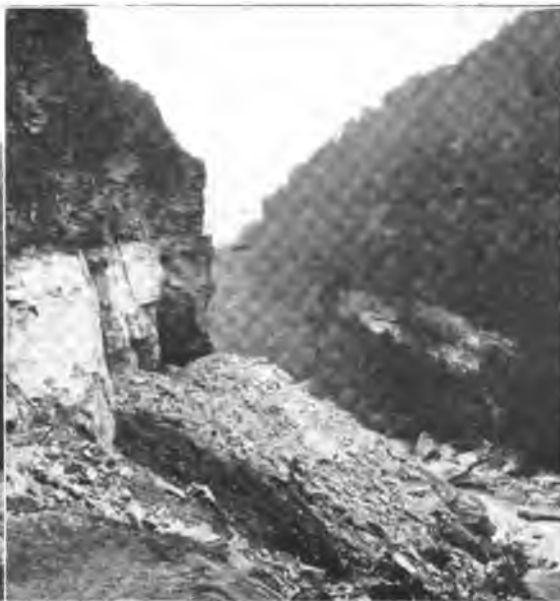
Benching Off Rock at "The Towers" Instead of Tunnelling.
