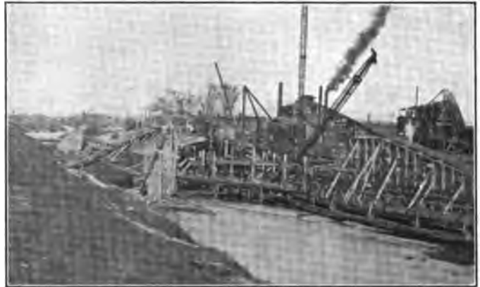
Building the Skew Arch Over the Present Erie Canal.
