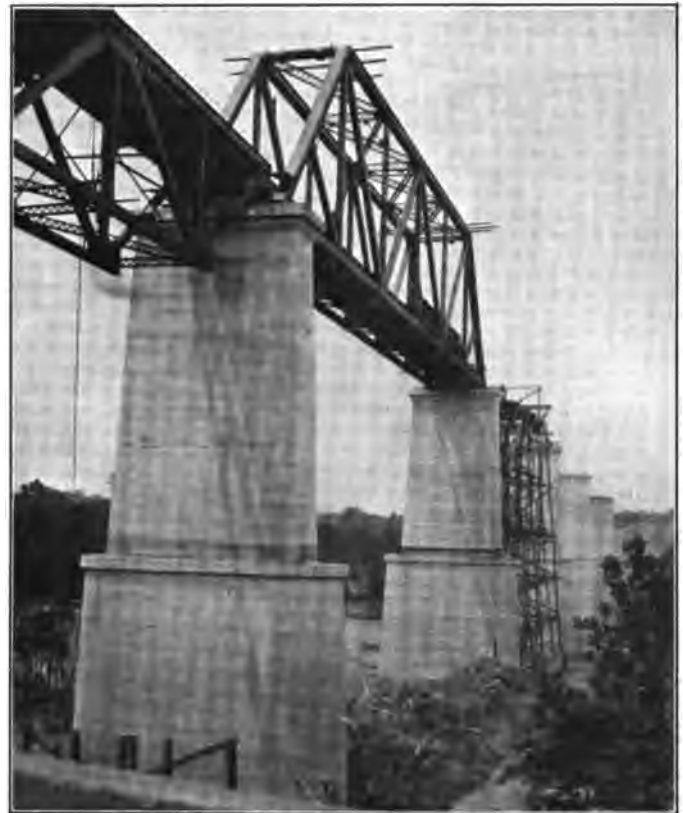
Cumberland River Bridge in an Early Stage of Erection.
