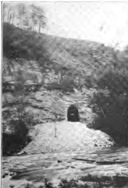
North Portal of Skag's Hole Tunnel.
