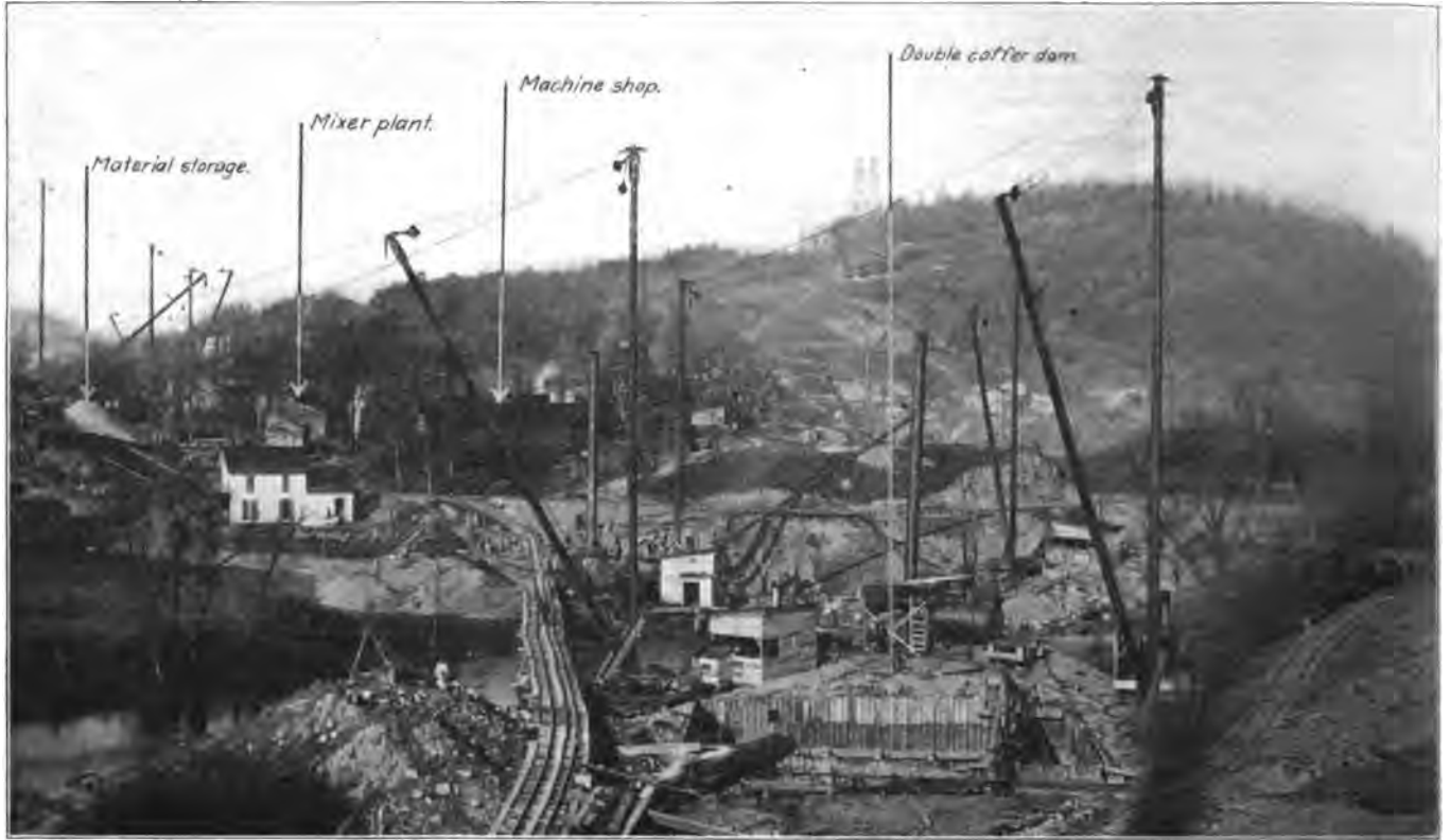
Looking Along Center Line of Tunkhannock Viaduct In Early Stages of Construction.
