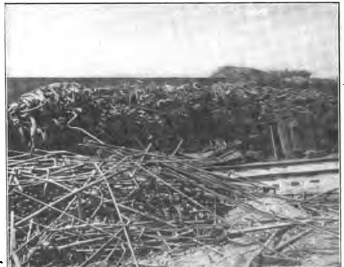
Fig. 9—Usable Material and Rods for Re-rolling Found in the Scrap Pile.
