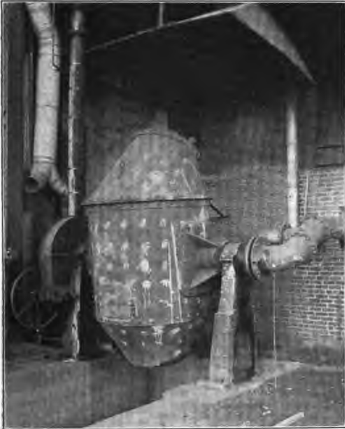
Side Blow Steel Converter of Two Tons Capacity.
