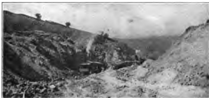
Shovel Removing 100,000 yd. Slide on Bear Creek Loop.
