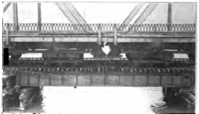
Trucks Carrying Bridge Over Deck Girder Falsework Span.
