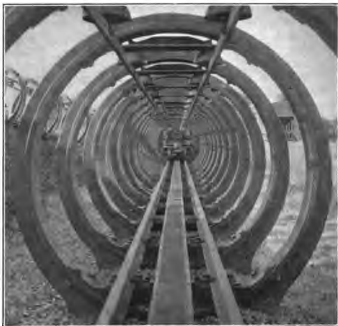
Arrangement of the Electric Carrier Within the Rings.
