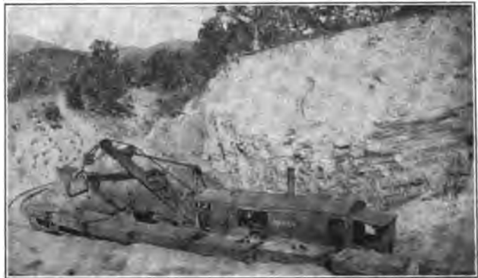
Shovel Working in Cut on Bear Creek Loop.
