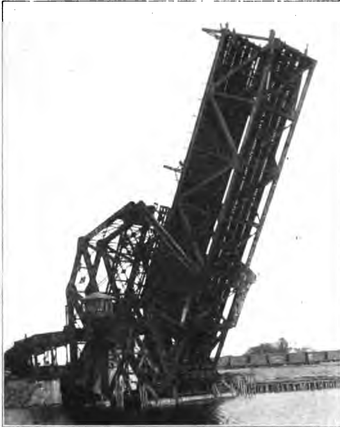
Fig. 5—Canadian Pacific Double Deck Bascule Span in Open Position.
