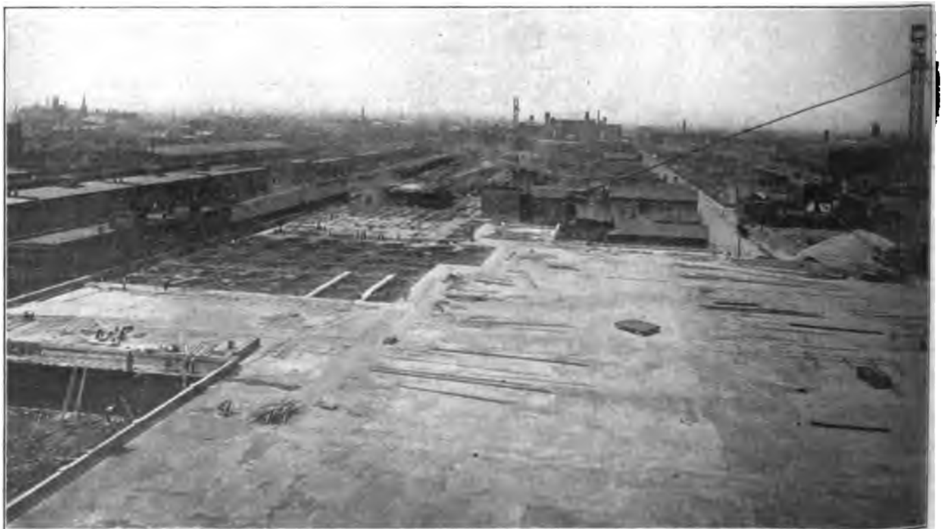
Surface of Track Slab Ready for Waterproofing.
