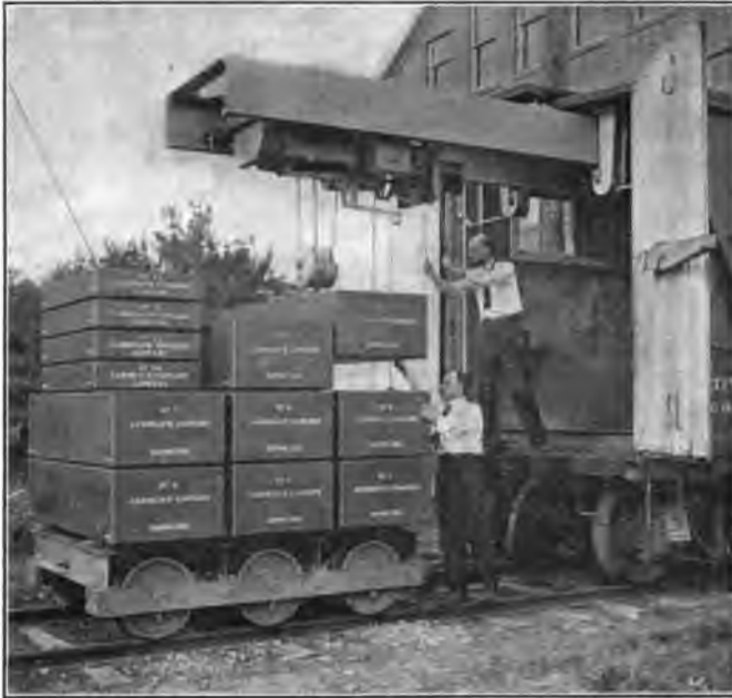
Truck, Standard Weights and Crane of Standard Scale Test Car.
