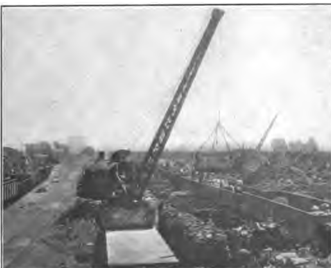
The pile just to the right of the flat car is usable material. Fig. 4—Method of Sorting Scrap from the Cars.
