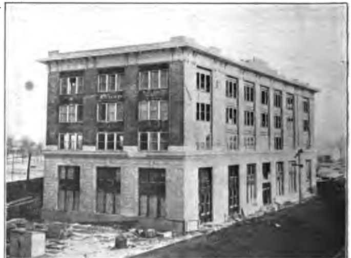
Station Building from Track Level, Looking Northeast.
