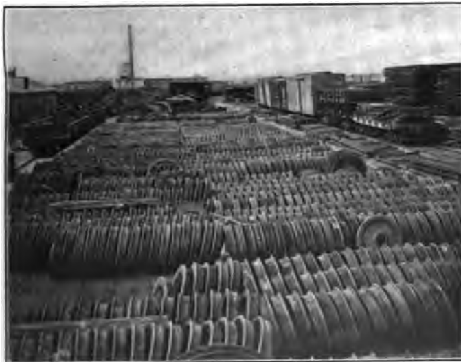
Fig. 7—Steel Wheel Centers Held for Re-tiring.
