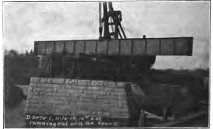
Carrying Girder for Brattleboro Bridge Out on Small Truck.
