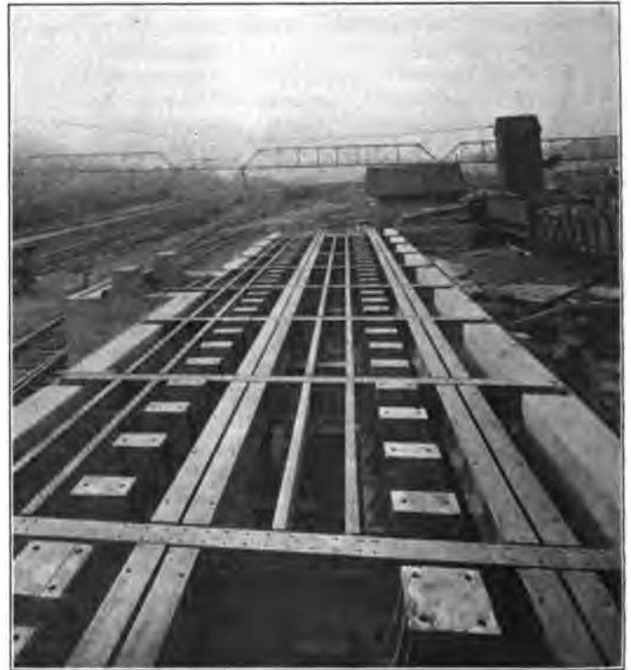
Fig. 4—Top of New Scale Ready for Application of the Deck.
