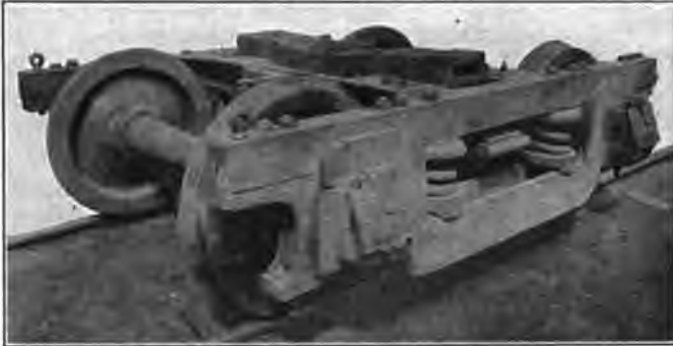
Equalized Tender Truck with Swing-Motion Bolster.
