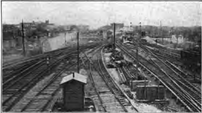
View Looking East from East End of Station Platforms, Showing High Retaining Wall on Left.
