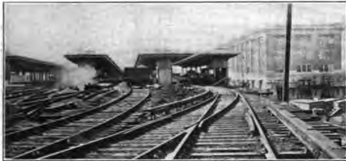
Station Building, Platforms and Shelters, Looking West.
