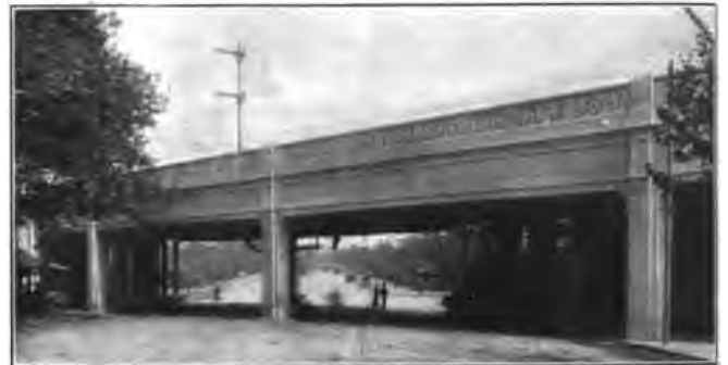
Steel Encased Bridge Over Girard Ave.
