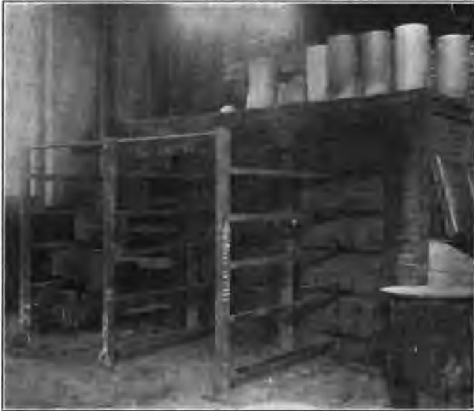
Battery of Drawer Type, Oil Fired Core Ovens.
