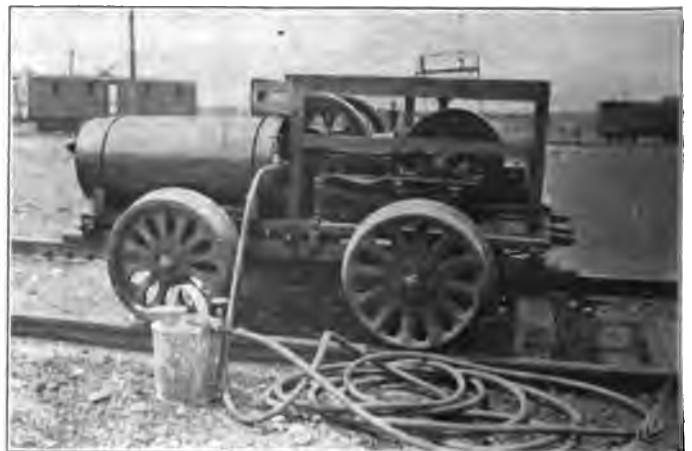
Compressor Plant on Motor Car for Spraying White Wash.
