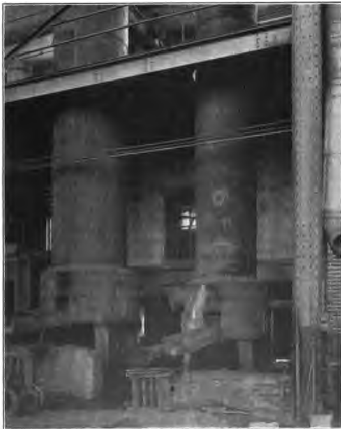
Arrangement of Cupolas in the Delaware & Hudson Foundry.
