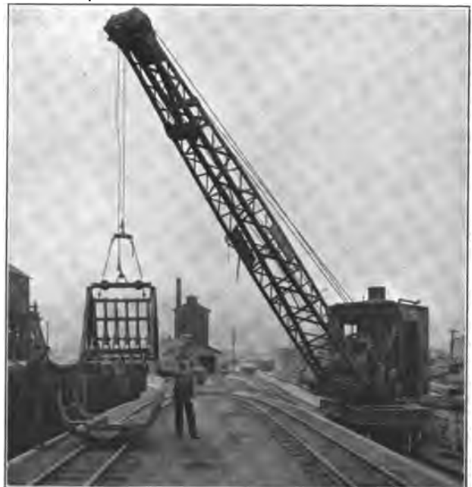
Tie Loading Device With Six Ties.
