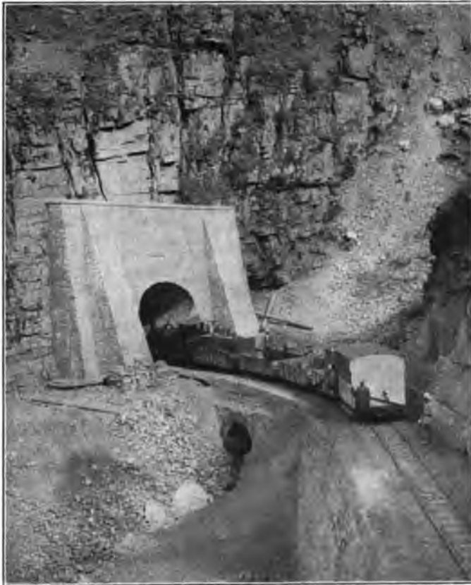
Difficult Tunnel Approach; Kalka-Simla Railway.
