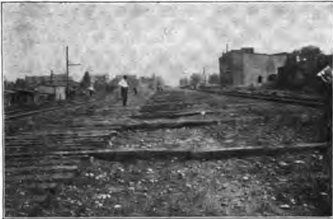
Preparations Completed for Lining Over Long Sections of Track.
