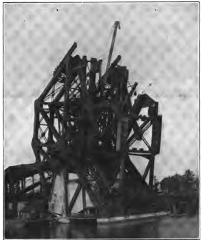
Fig. 3—Erecting Double Deck Bascule Bridge in Open Position.
