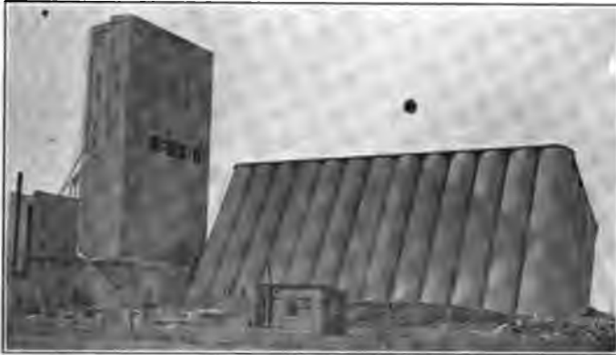
View of Inclined Bin and Undamaged Headhouse.
