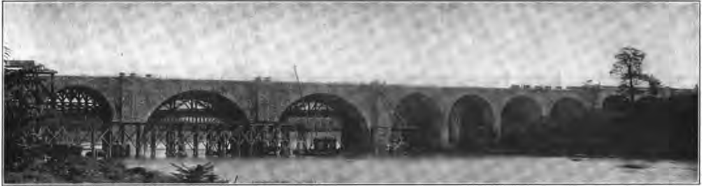
Double-Track Addition to Schuylkill River Bridge Before Placing Railing.
