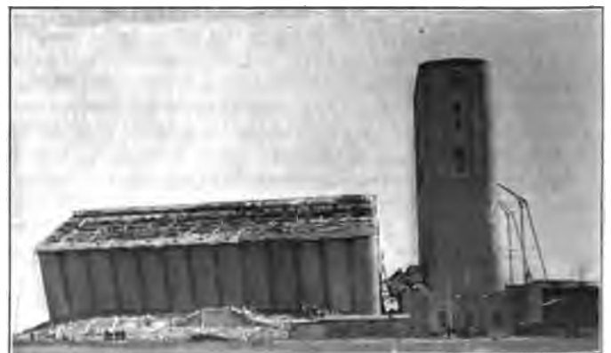
Looking Toward Inclined Bin After Roof Had Slid Off.
