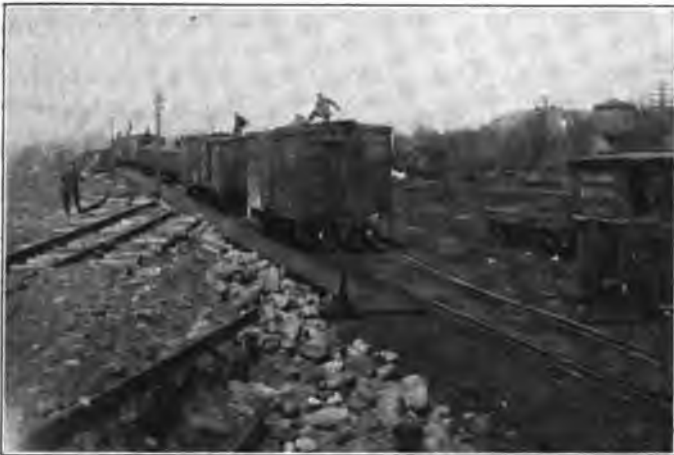
Temporary Hump in Operation.
