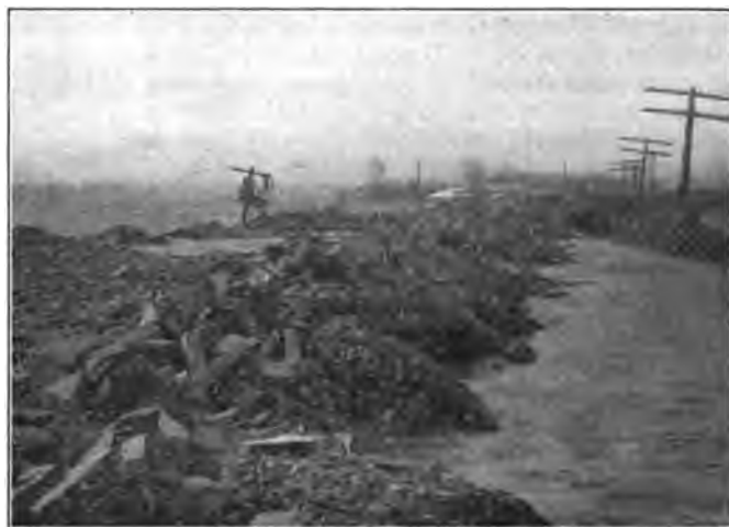
Fig. 3—Condition of Roadbed After the Flood at the Wabash River Crossing near Lafayette, Ind.—Ties Standing on End Against Telegraph Poles.
