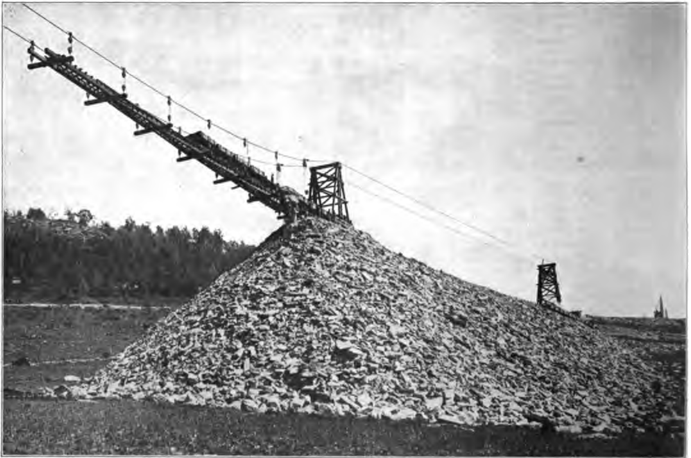
One End of Cableway at Riker Fill, Showing Movable Intermediate Tower.
