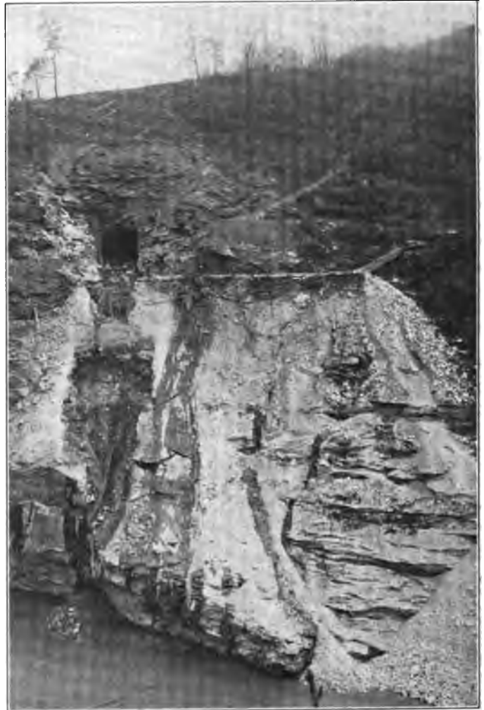
Pool Point Looking Across River Toward North.
