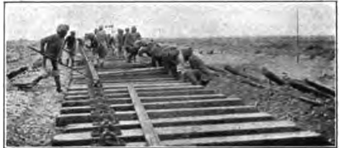
Turning the Rail Over in the Chairs.
