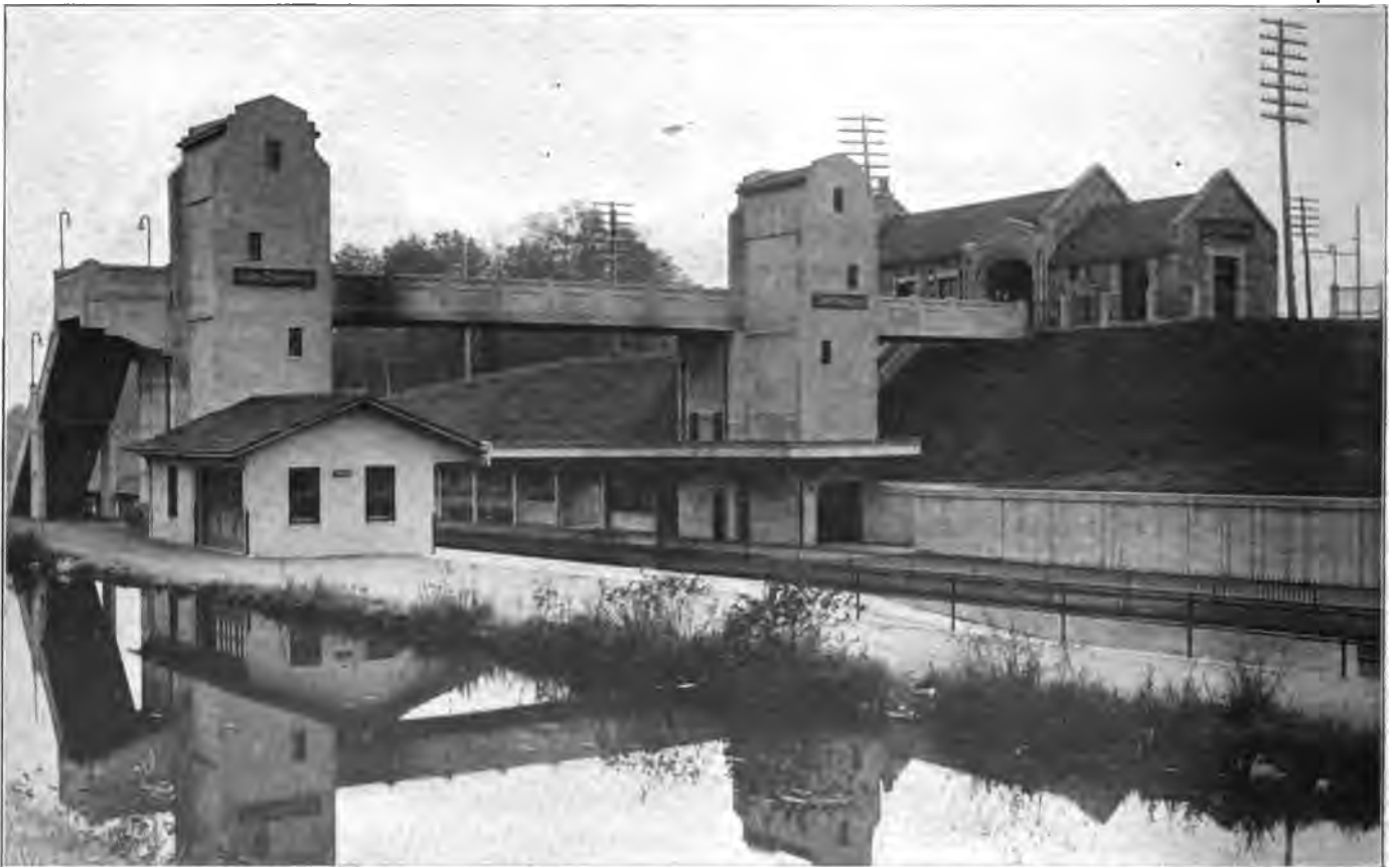
Novel Station of Concrete and Cobble Stones at Lake Hopatcong, N. J.
