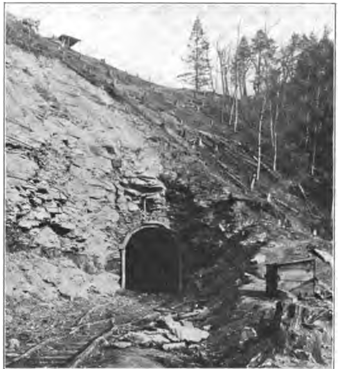
South End of Caney Creek Tunnel, Which Was Driven by Hand.
