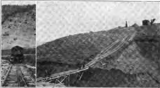
Moving a Steam Shovel Up a Forty Per Cent. Incline.
