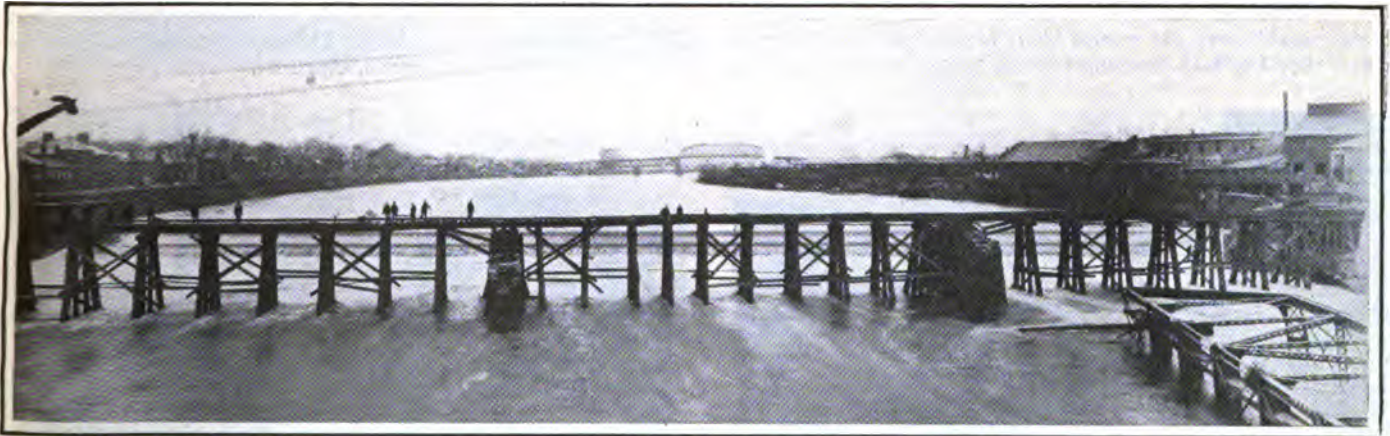
The Crossing Completed at Zanesville After One Week's Work.
