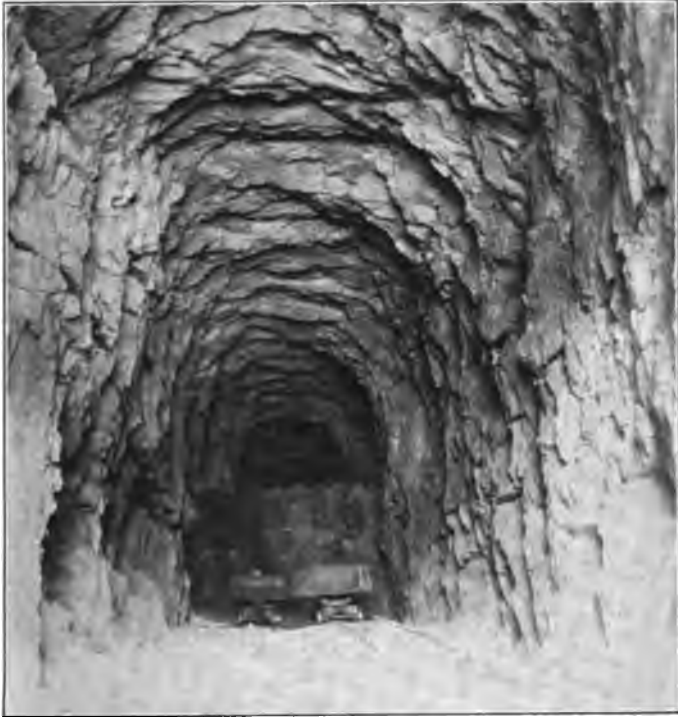
Skag's Hole Tunnel.
