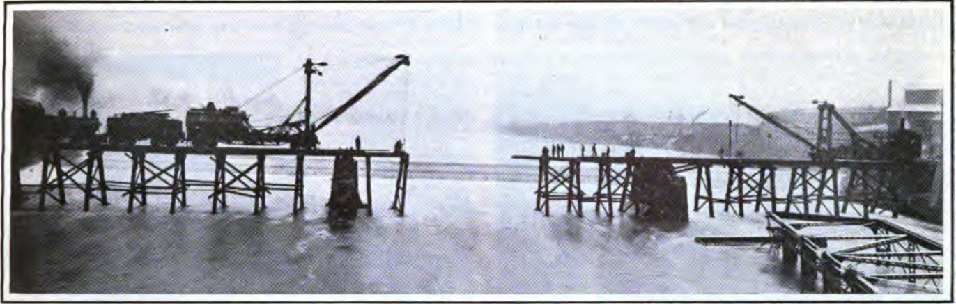
At Work on the Reconstruction of the Zanesville Bridge.
