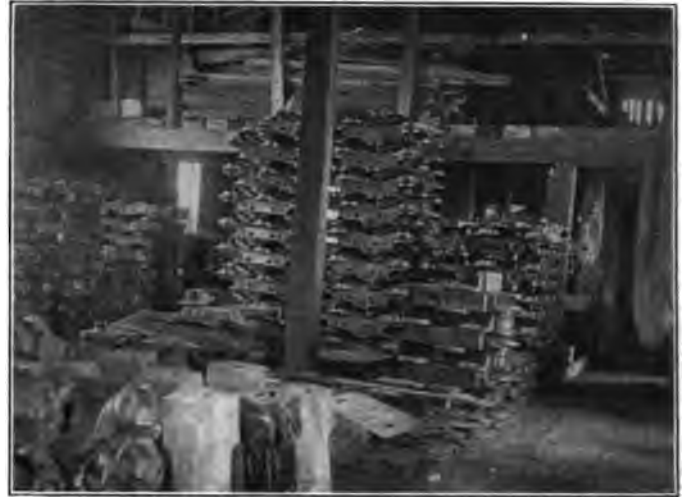
Fig. 16—Interior of the Storehouse for Reclaimed Material.
