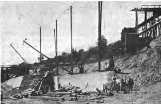
Contractor's Layout for Arch Under Smith Fill.
