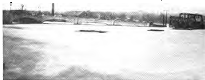
Three Spans Gone at Zanesville.
