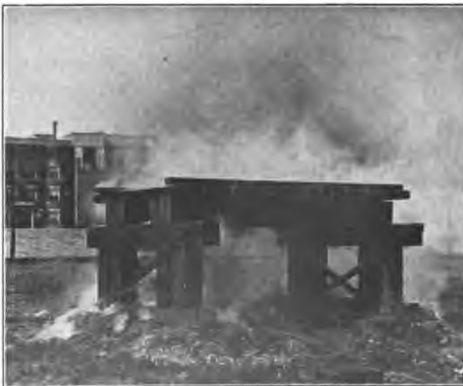
Effect of Fire on Test Trestle at Chicago; Surface Charred Only.
