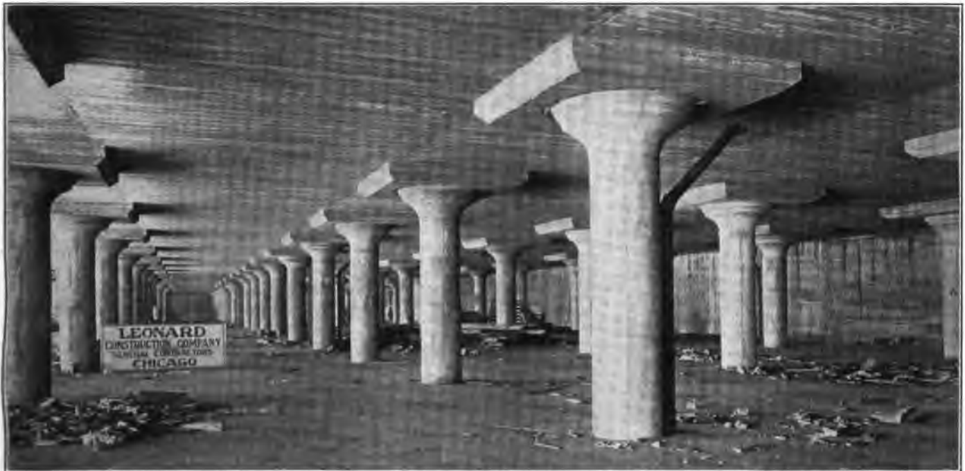
View Under Track Slab Showing Typical Construction.
