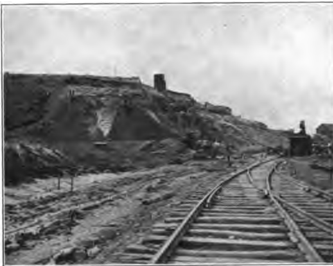
Terracing Slope in Sliding Cut.
