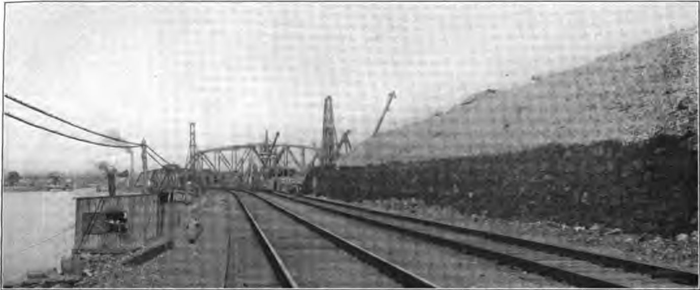
Stone Cribbing Along 20-ft. Fill for New Line.
