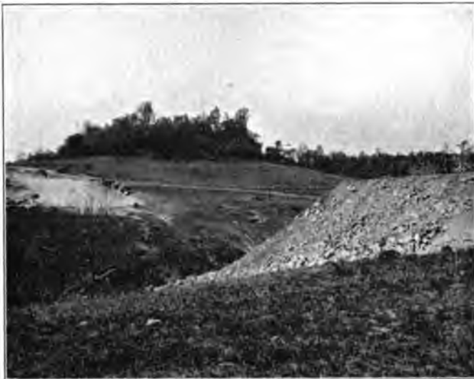
Making a High Fill with a Cableway.
