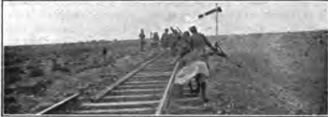
Dismantling the Old Road.
