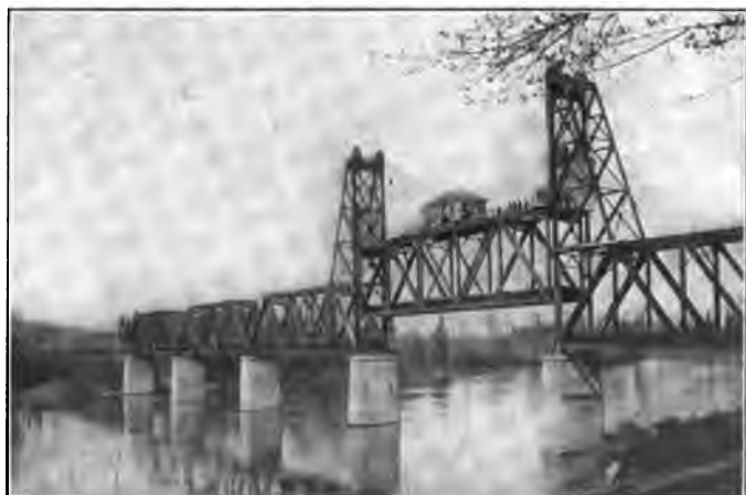
Recently Completed Bridge Across the Willamette River at Salem, Ore.
