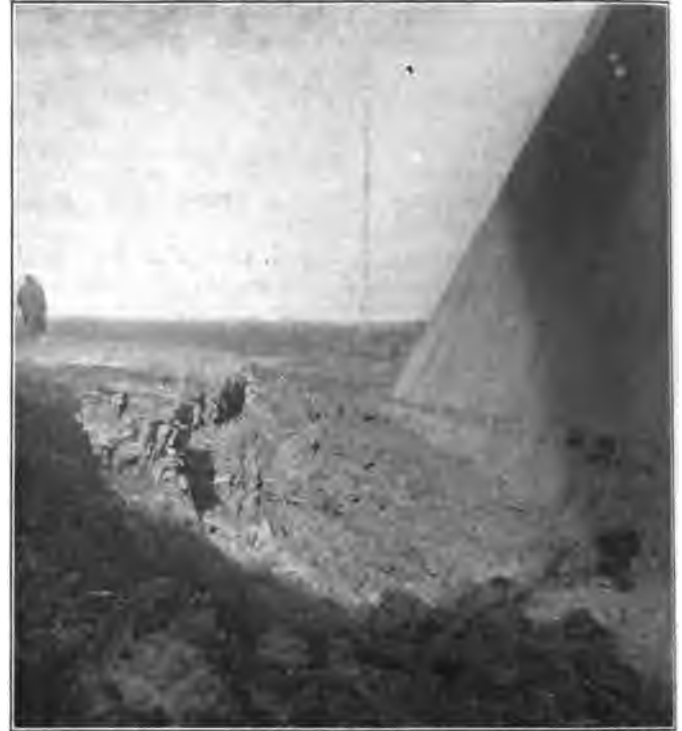
Breaking of Ground Surface on Upper Side of Elevation.
