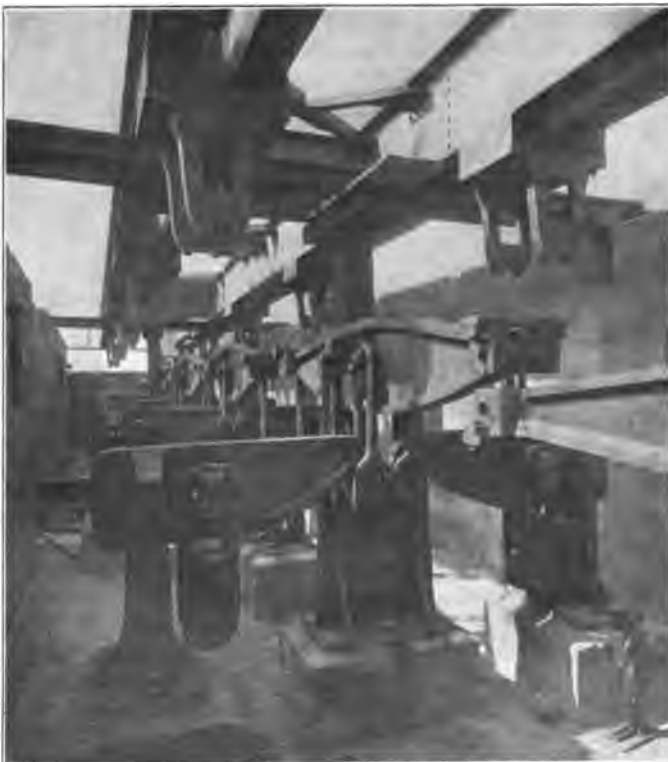
Fig. 3—Construction View of New P. & L. E. Scale.
