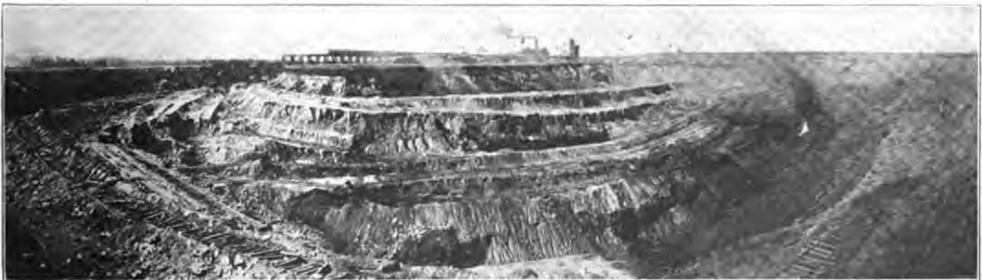
Fig. 3—An Illustration of the Number of Levels in an Open Pit Mine in the Missabe District.
