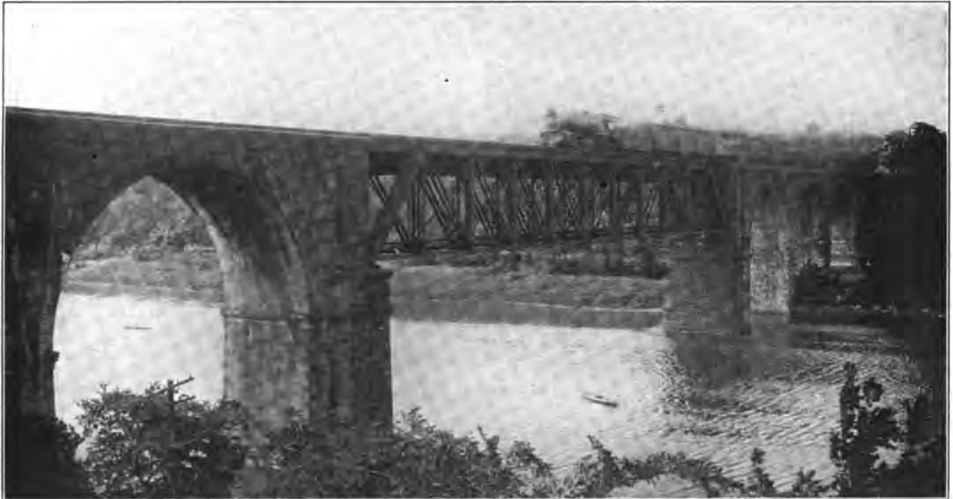
General View of Old Bridge.
