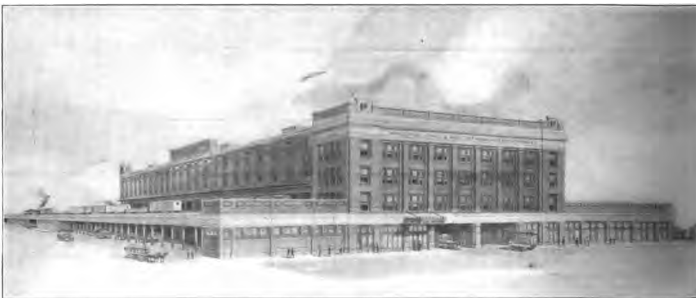
Perspective of Freight Buildings Facing Twelfth Street As They Are Being Built.
