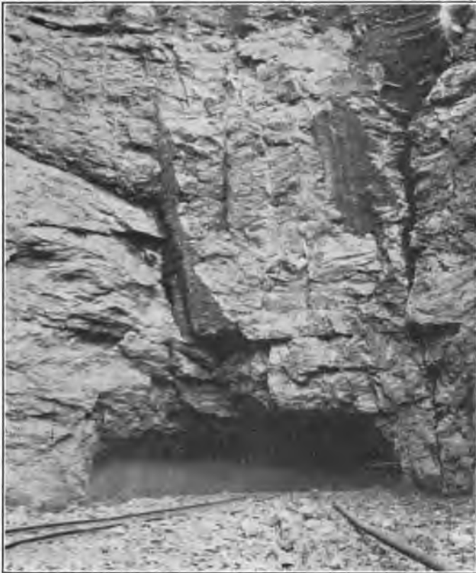
Bottom Heading in Rock Tunnel Near Blount Springs.
