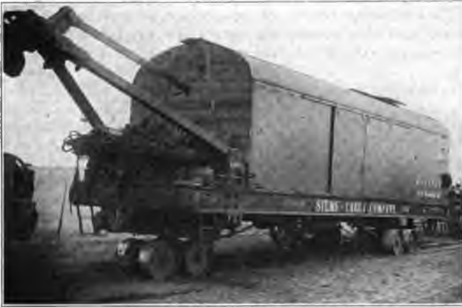
Steam Shovel Mounted on Trucks Ready for Moving.
