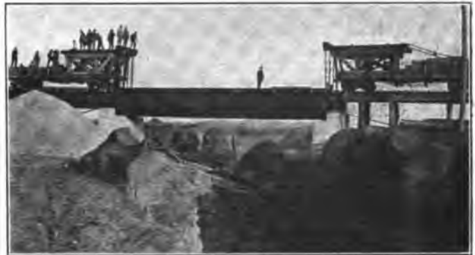
Girder Loaded Into Position.
