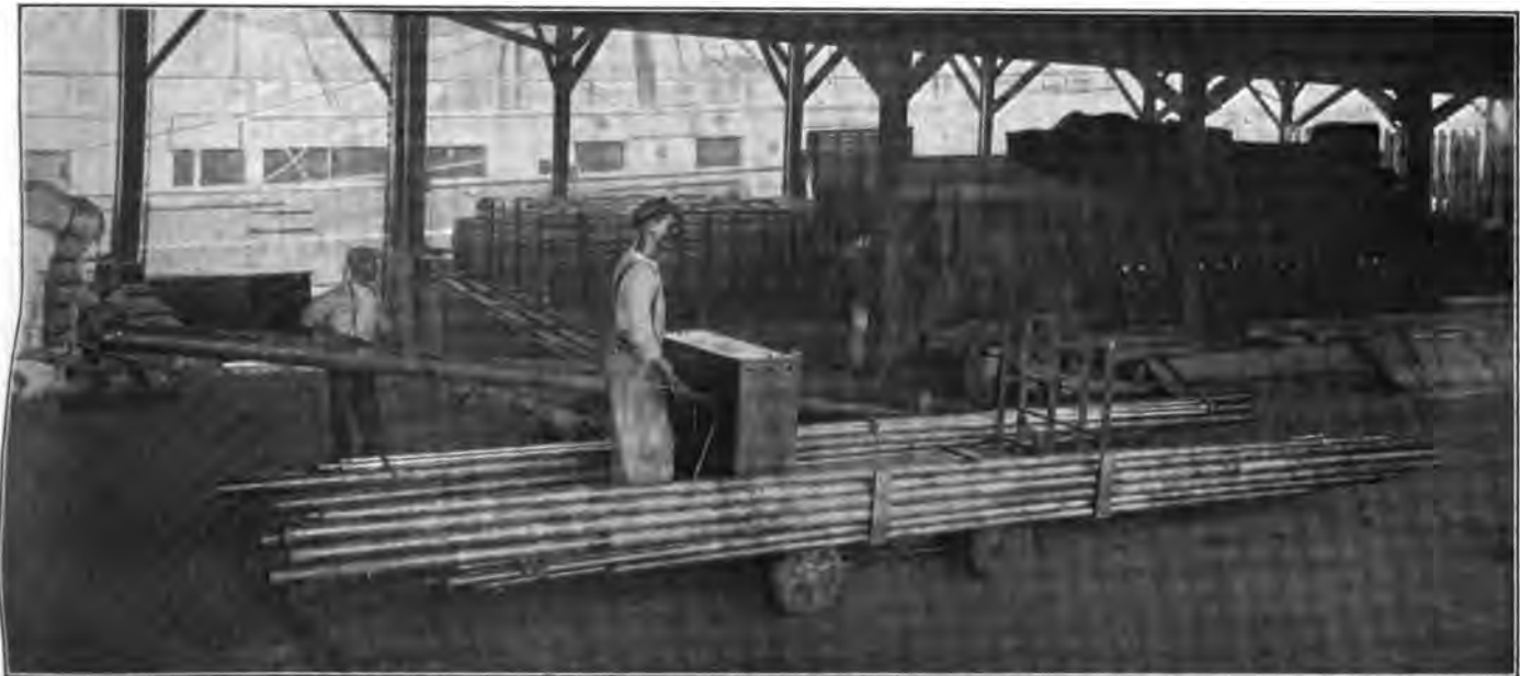
Truck Carrying Pipes on Pier of the Merchants' & Miners' Transportation Company, Savannah, Ga.
