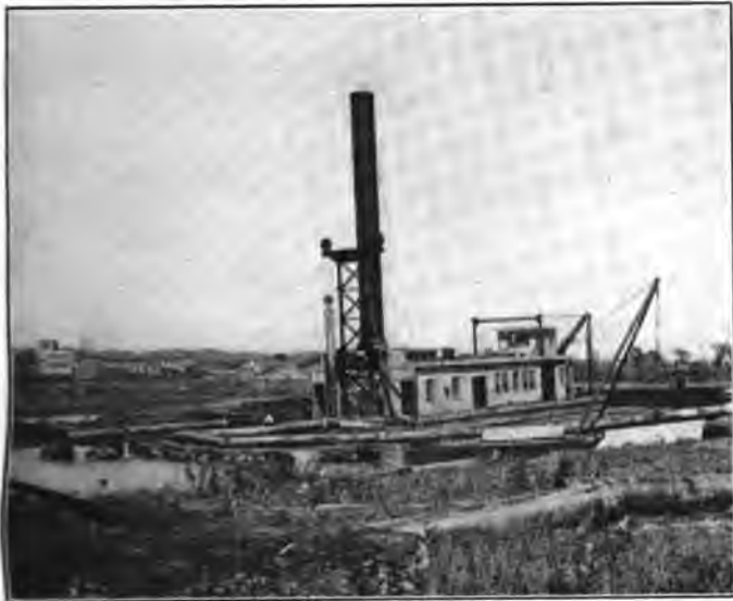
Hydraulic Dredge Working in New Barge Canal South of Rome, N. Y.
