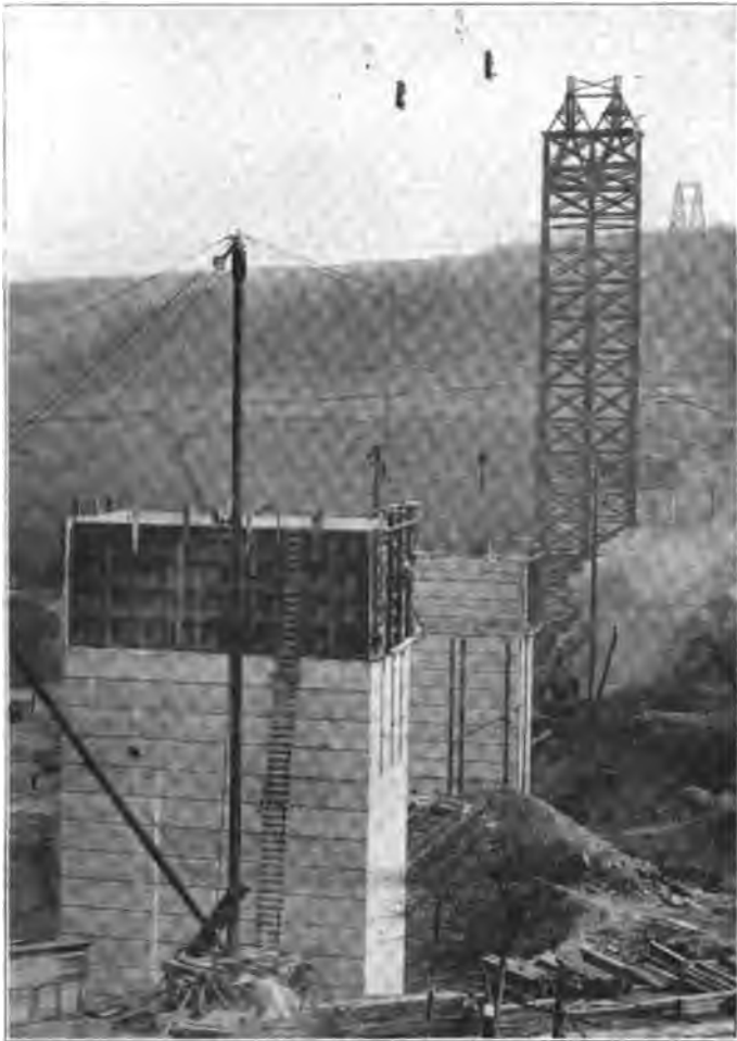
Showing Sectional Pier Forms and Double Cableway.
