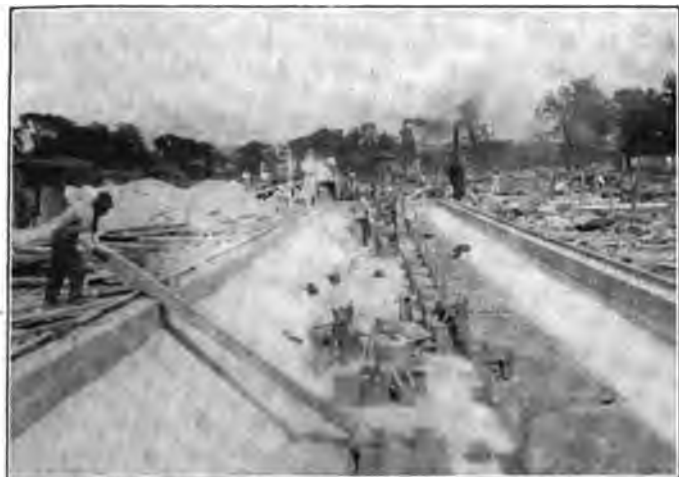
Laying the Firebrick Lining in the Ash Pit.
