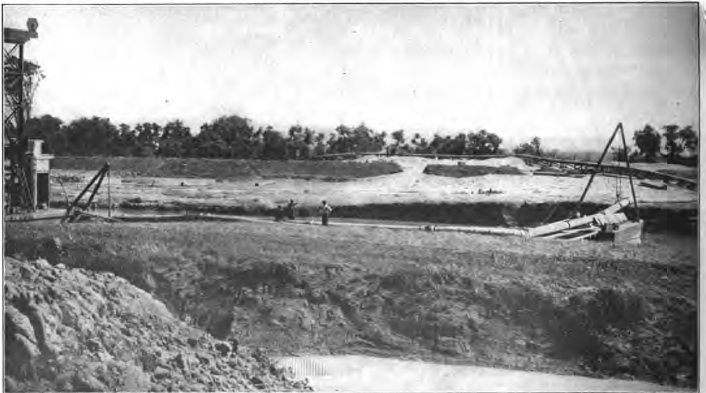
Discharge Pipe and New Embankment Being Made by Dredge.
