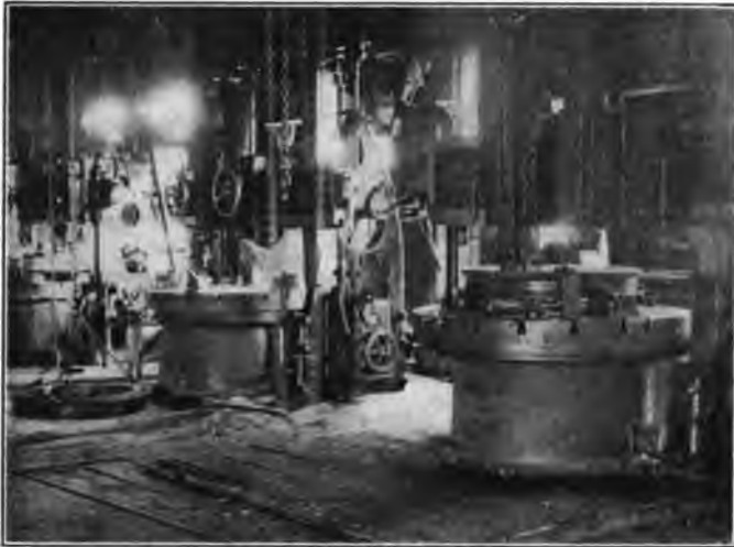
Fig. 15—Boring Mills in the Wheel Shop.
