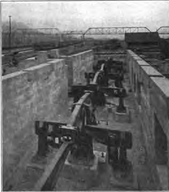
Fig. 2—Arrangement of Levers of New P. & L. E. Scale in Pittsburgh.
