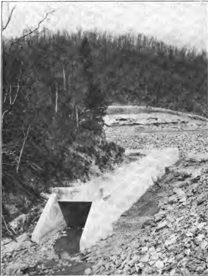
Long Concrete Culvert near Dante.
