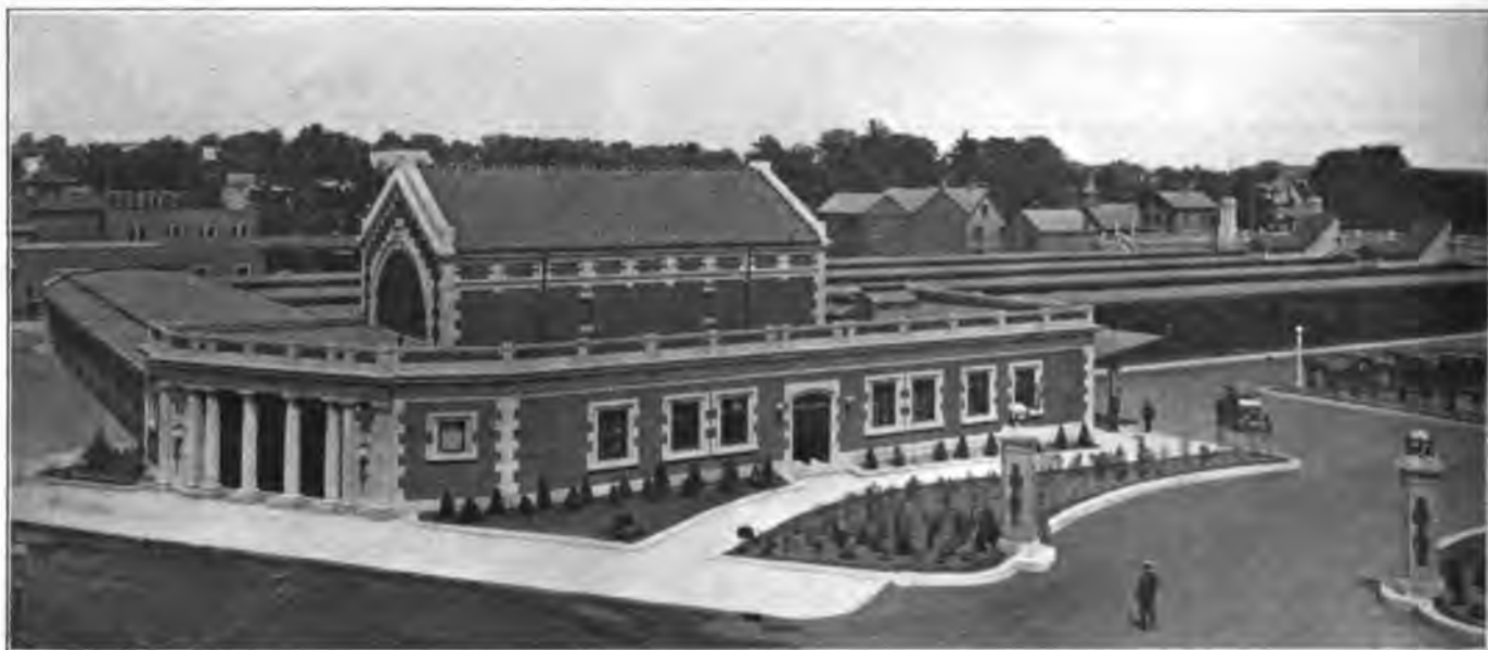
General View of Montclair Station and Trainshed.
