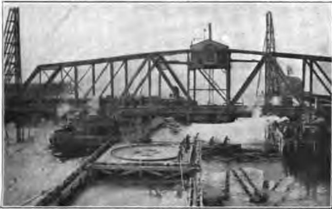
Moving Old Hackensack Draw Span to Temporary Position.
