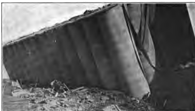
Closer View of Under Side of Bins.
