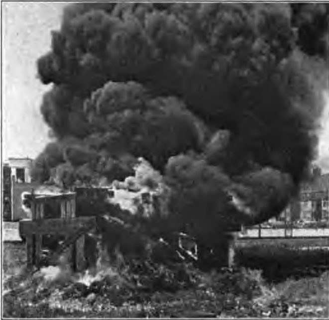
Attempting to Burn a Section of Test Trestle at Chicago.
