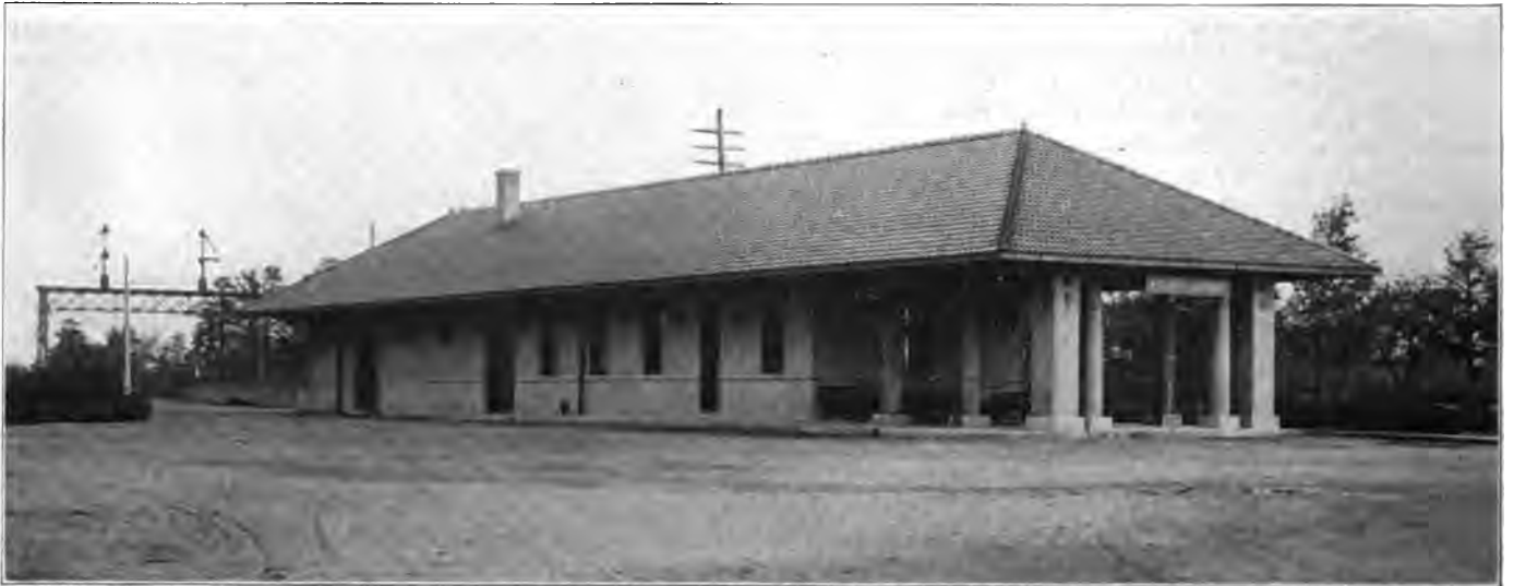
Concrete Station at Pocono Summit, N. J.
