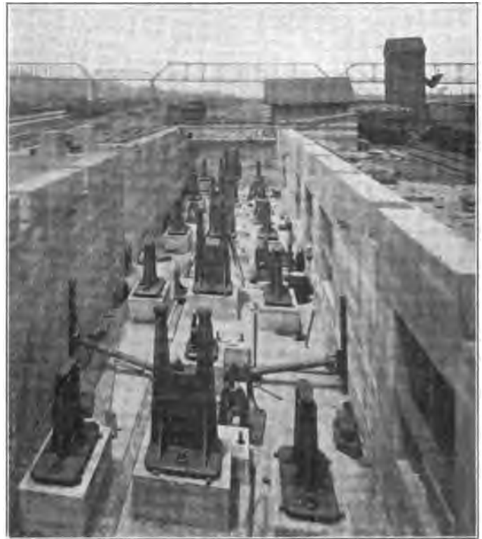
Fig. 1—Pedestals in Place in New P. & L. E. Scale.
