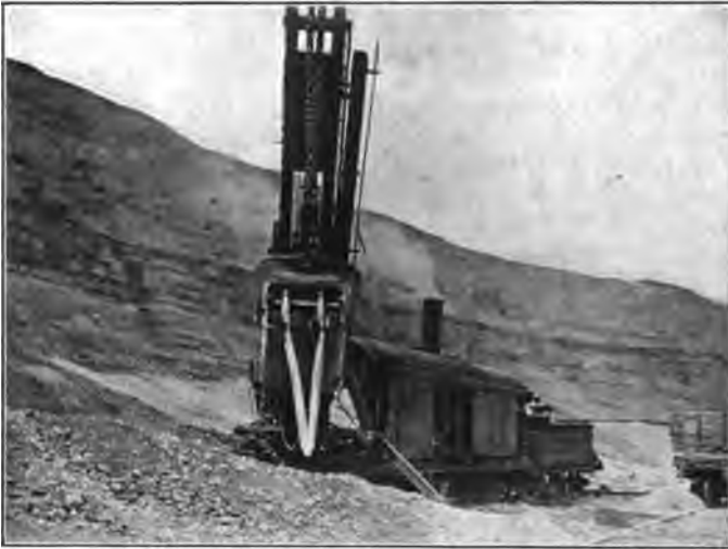
Attachment in Position on Shovel Dipper.
