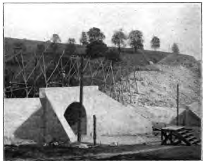
Typical Culvert Construction.
