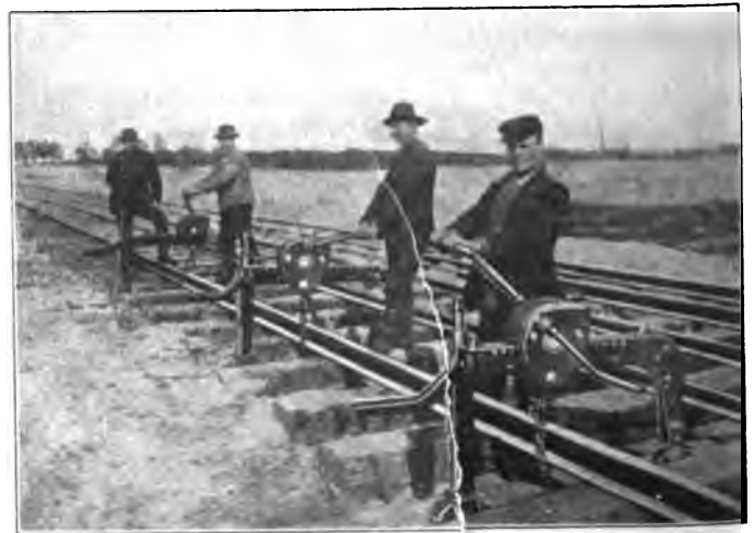
Track Shifters in Operation.
