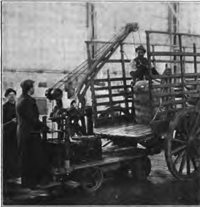
Truck Crane of One-Ton Capacity.
