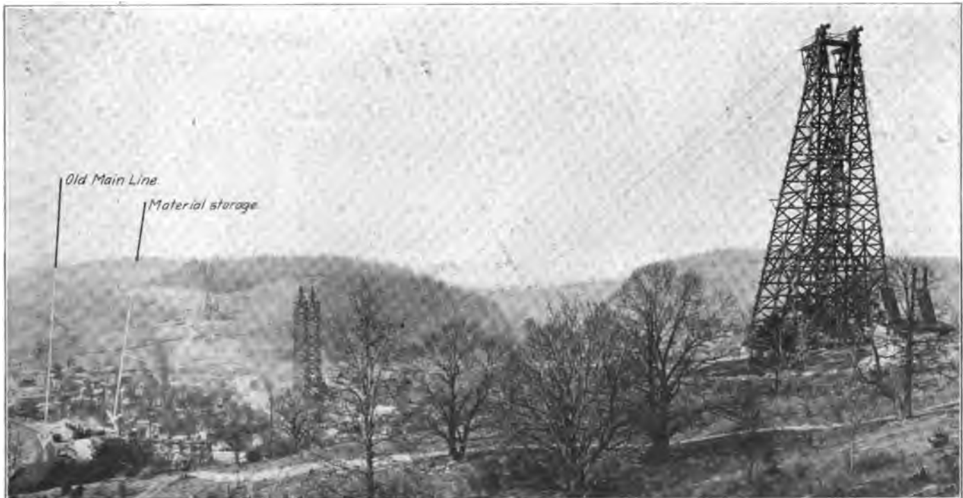
General View of Tunkhannock Viaduct Location, Showing End Tower and Operator's House of Material Cableway in Foreground
