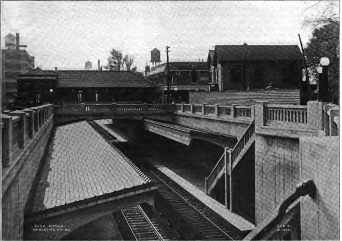
Brick Station with Concrete Trimmings at Watessing Ave., N. J., Showing Concrete Cantilevered Canopies.
