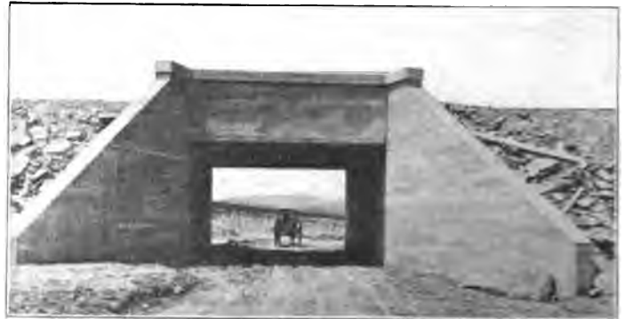
A Typical Highway Undercrossing.
