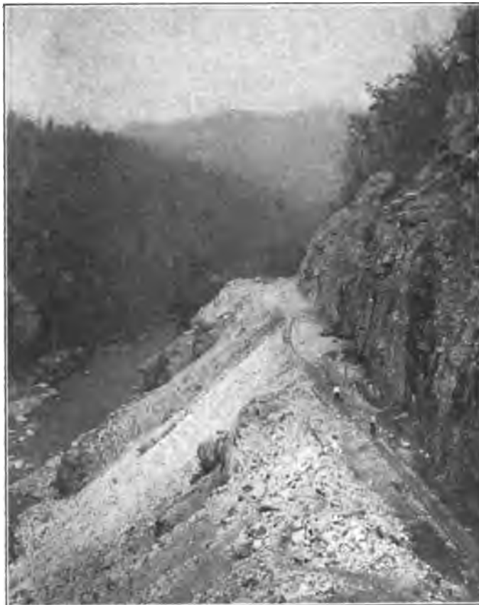
Looking North from Top of Pool Point Tunnel.
