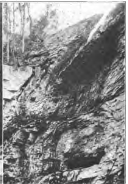
North Heading of Towers Tunnel.
