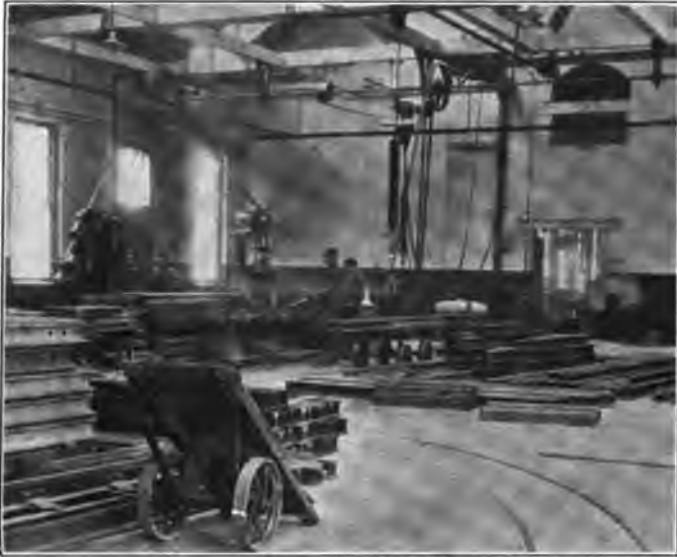
View of Switch Assembling Room.
