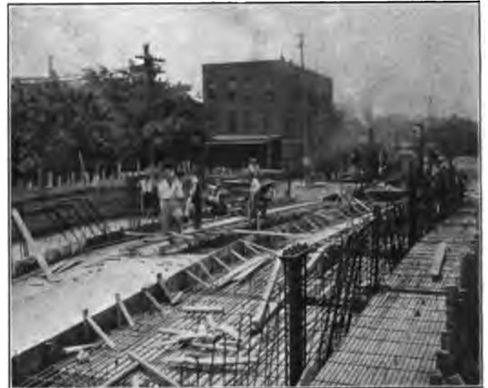
Reinforcement and Contractors' Plant for One of the Cullman Viaducts.
