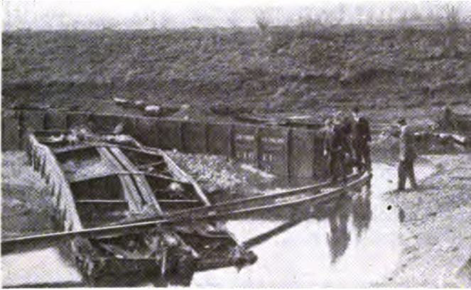
One Example of the Flood Damage near Dayton, O.
