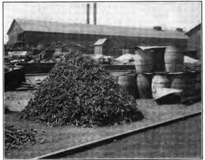
Fig. 8—Track Spikes and Barrels of Nuts to Be Reclaimed.
