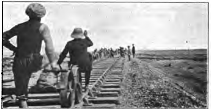
Straightening the New Road.
