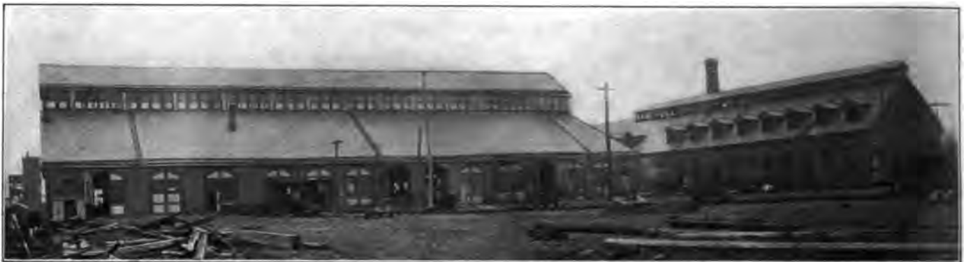
Exterior of Frog and Switch Shop Before Old Debris Was Cleared Away.
