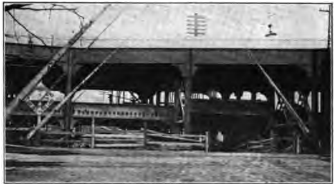
Van Wyck Avenue Bridge, from Roadway, Looking North.
