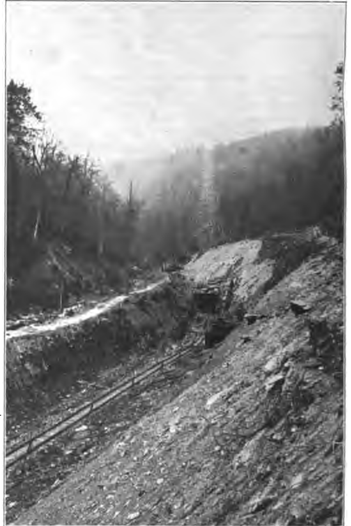
South End of Sandy Ridge Tunnel.
