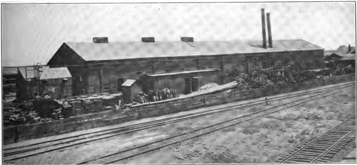
Fig. 1—Main Shops for Reclaiming Scrap at Corwith, Ill.; Atchison, Topeka & Santa Fe.
