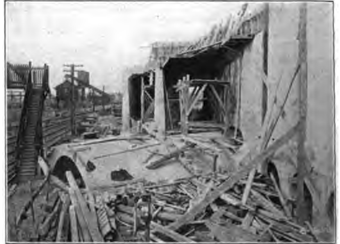
Maure Avenue Underjump Under Construction, Looking West.
