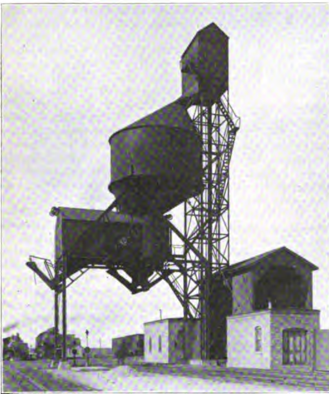
New Coaling Station and Sand Handling Plant at Minidoka, Idaho.
