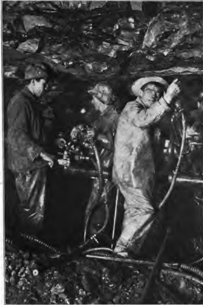
Fig. 5—Heading Where Record Progress Was Made, Showing Water Connection to Drills.
