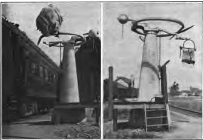
Fig. 3—A Bag That Has Been Taken from a Train. Fig. 4—Bag Waiting for Train.
