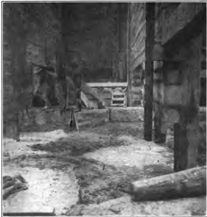
Laying Masonry in Caisson of North Main Pier.
