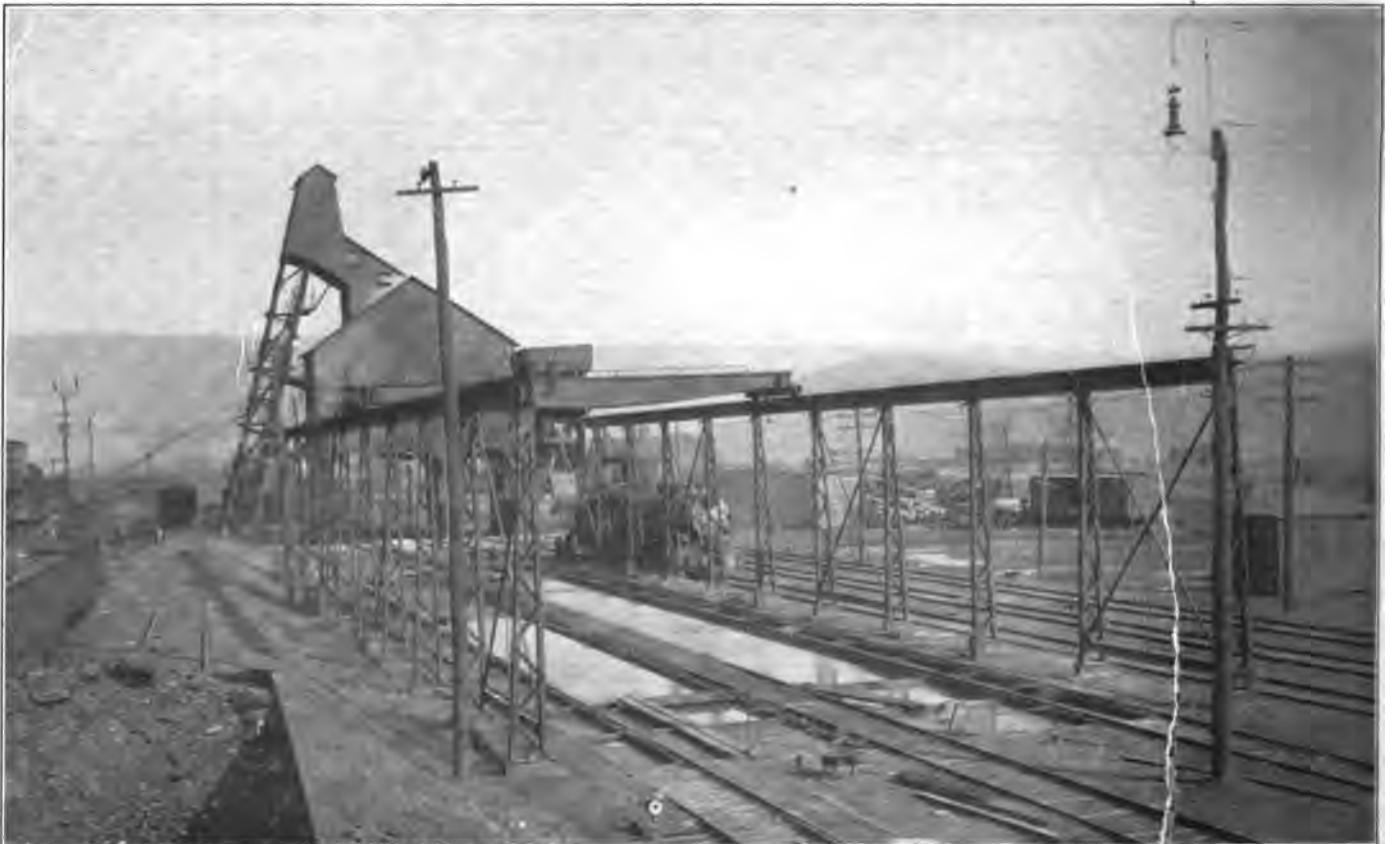
Clinker Pit and Coaling Station.
