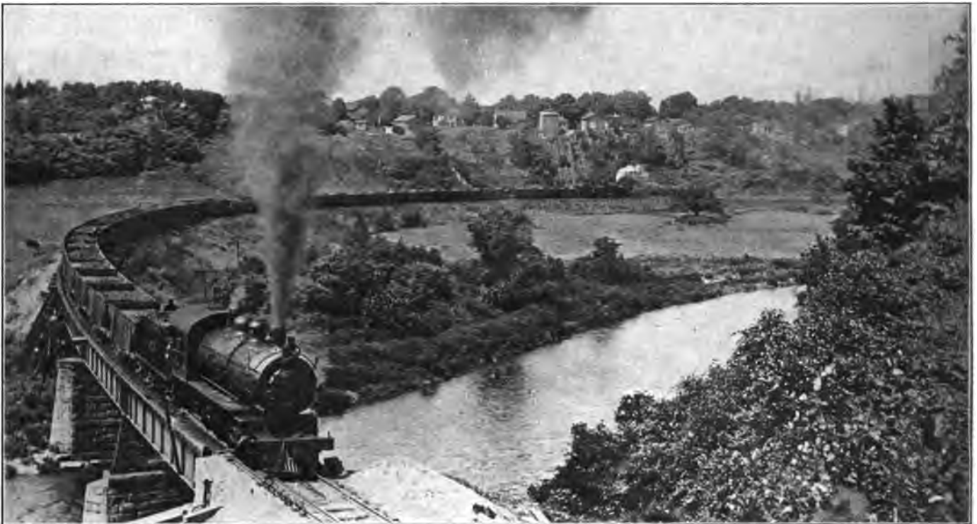
Fig. 7—Typical Ore Train of the Bessemer Road Leaving Conneaut Harbor.
