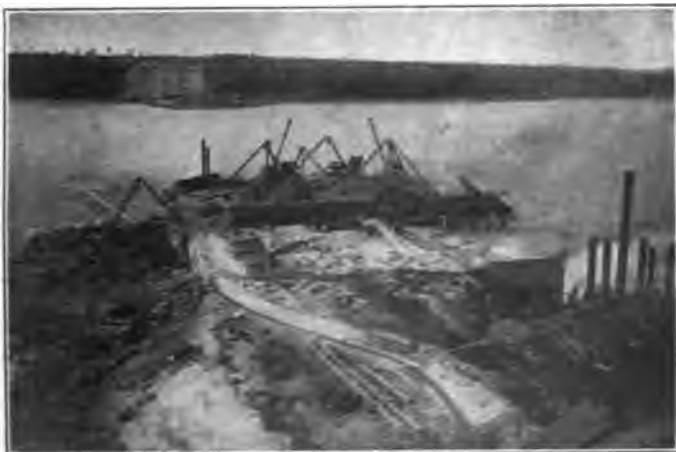
General View of Plant on South Shore.
