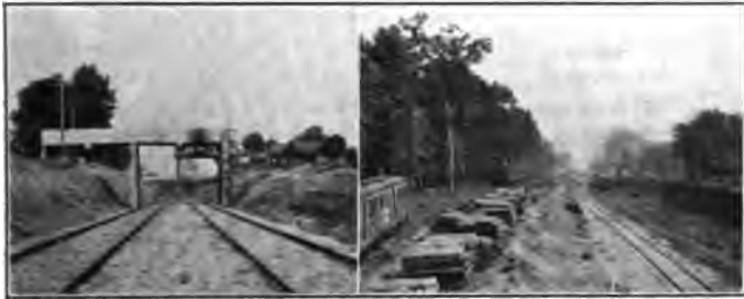
Cullman Cut Showing Via-ducts. A Typical Piece of Company Work.
