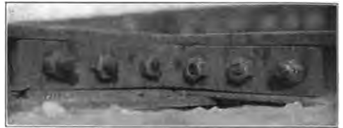
Absolute Lock Nuts on an Illinois Northern Crossing.
