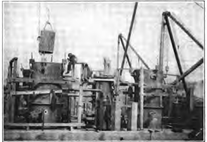
Service and Ladder Shafts of Caisson at North Main Pier.
