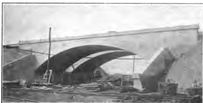
Double Concrete Arch Structure Over Avenue R.
