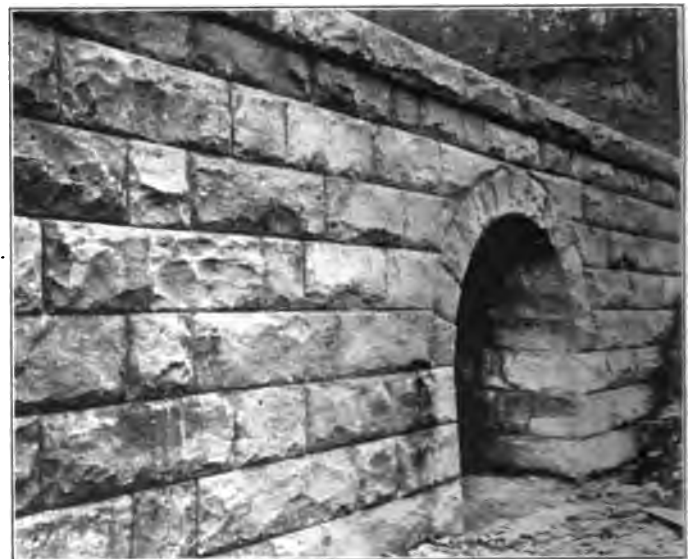
Spring Branch Stone Headwall.
