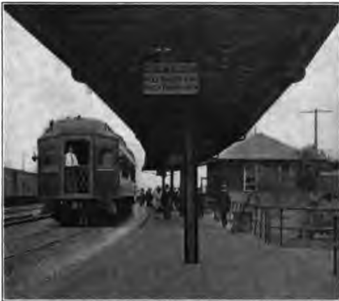
Safety Sign and Line at Englewood Station, Chicago.
