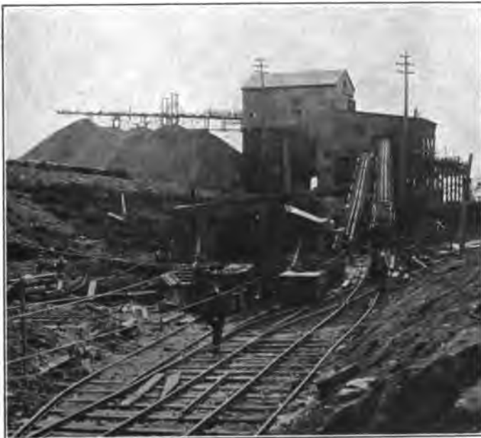
Fig. 3—Crusher Plant and Tipple at West Portal.
