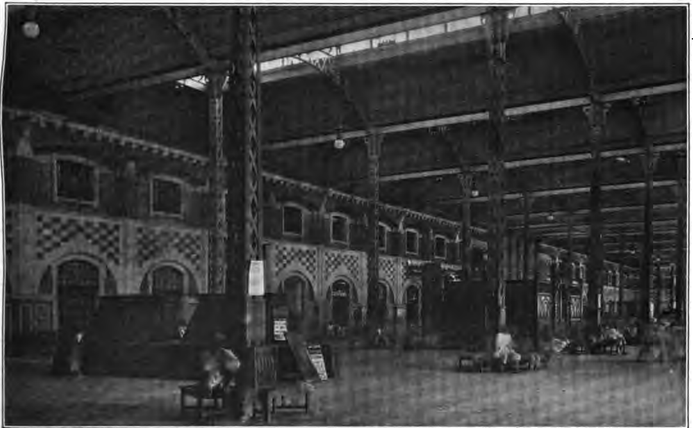
Interior of the E. I. R. Station at Calcutta, the Largest Station in India.
