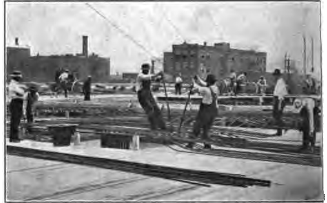
Bending Slab Reinforcement in Place.
