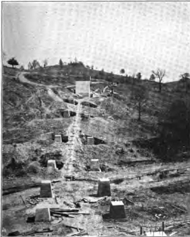
Footings and Abutment for Dry Fork Viaduct.
