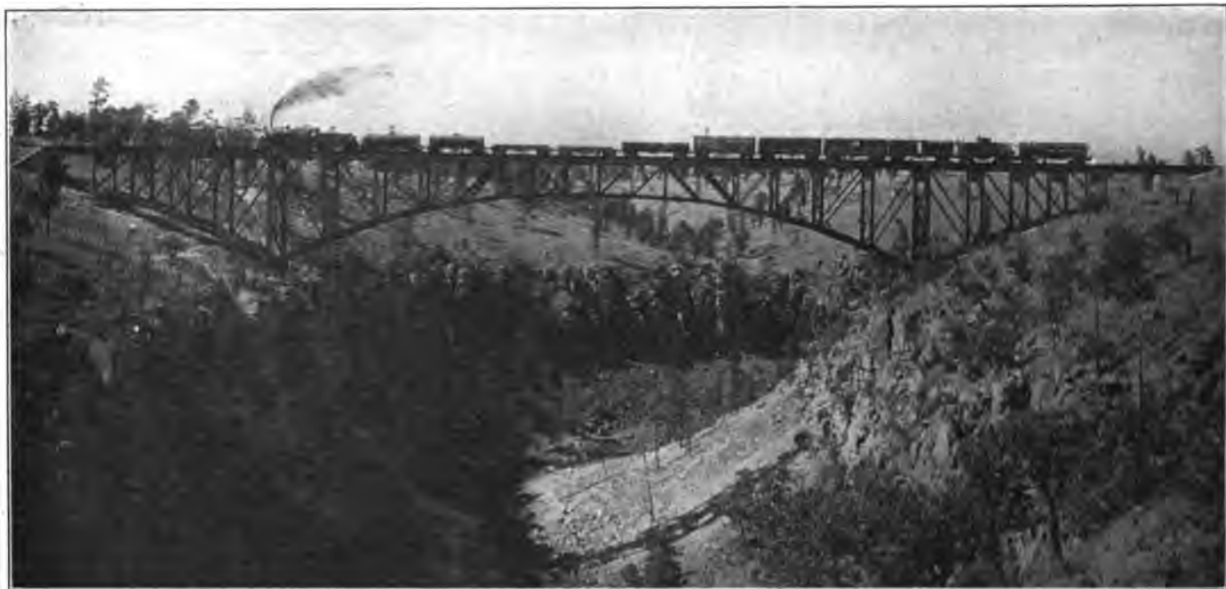
The Completed Structure in Service.
