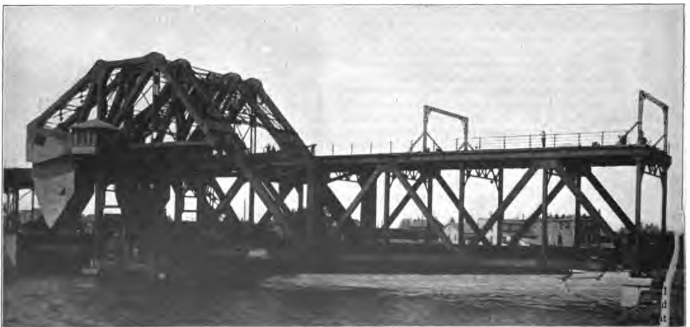
Fig. 4—New Double Deck Strauss Bascule Span over Kaministiquia River.
