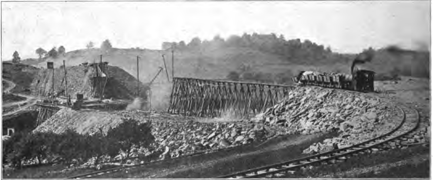
Smith Fill, Showing Balanced Incline and Second Level Dumping Trestle.
