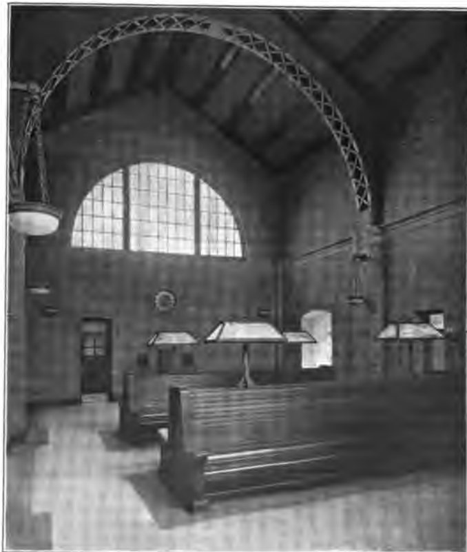
Interior of Waiting Room, Montclair Station.
