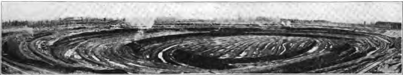
Fig. 2—A Typical Pit in the Missabe District with Circular Approach.
