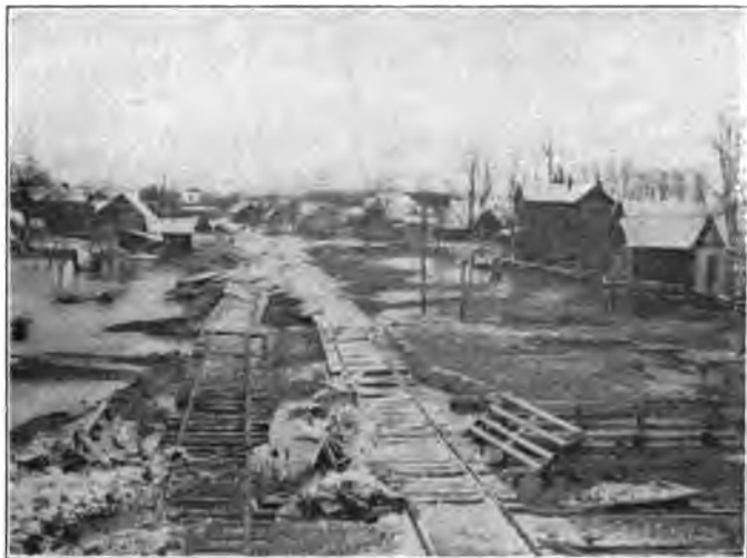
Fig. 1—Monon Tracks in Broad Ripple, Ind., After the Flood Had Partially Subsided.
