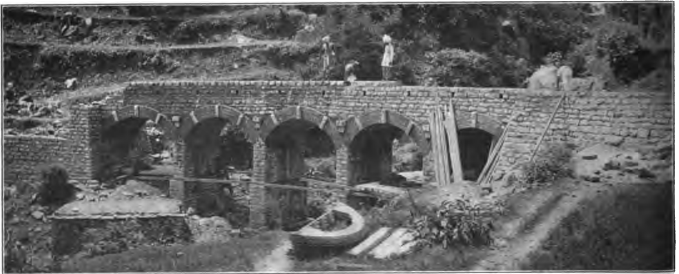
Type of Bridge Construction; Kalka-Simla Railway.
