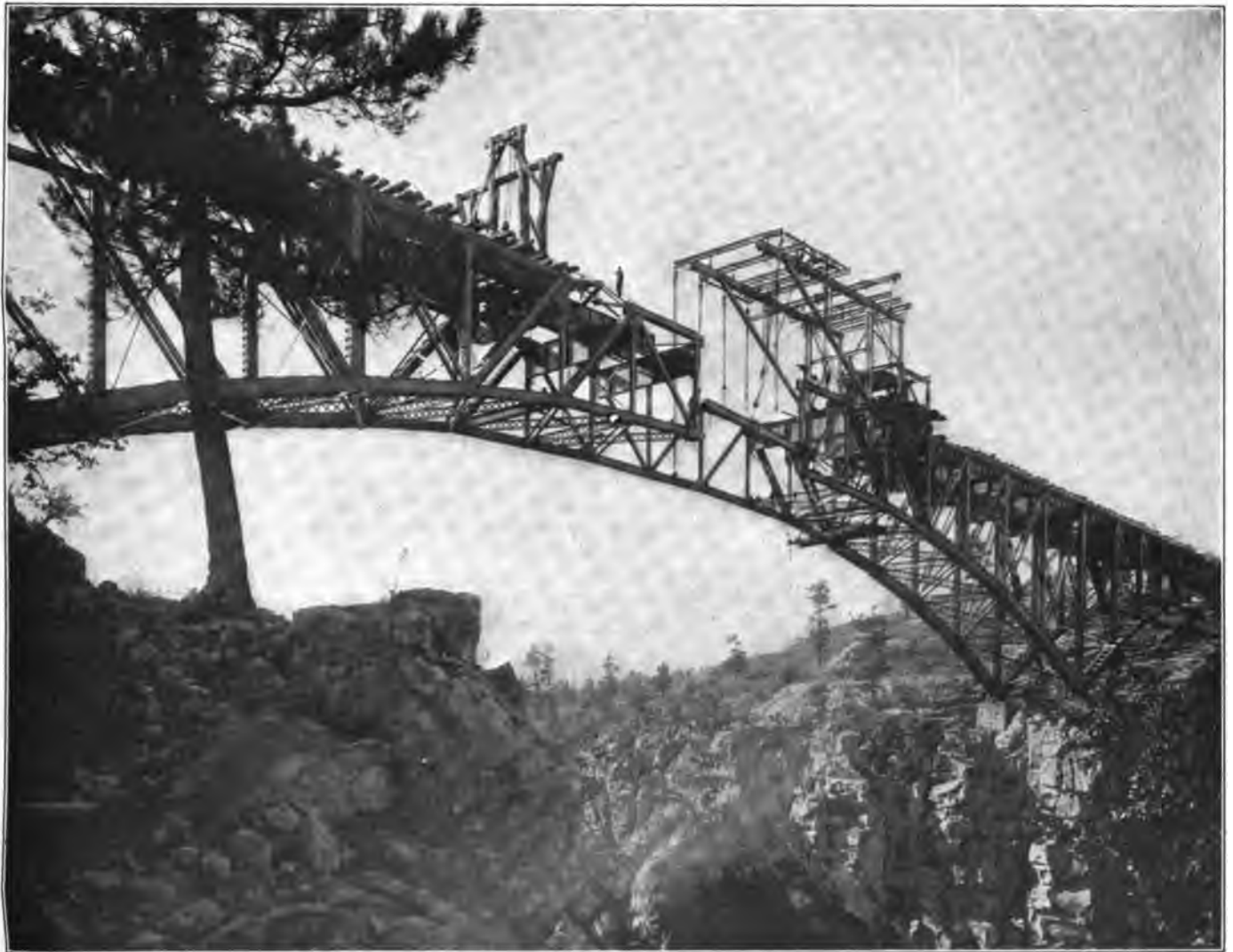
Placing Last Section of Lower Chord.
