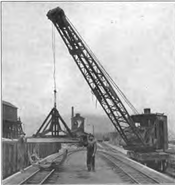
Side View of Tie Loading Device.
