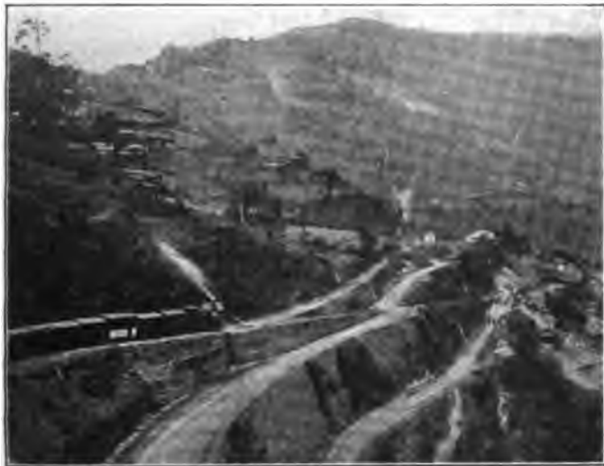
Switchback on the Darjeeling Himalayan Railway.
