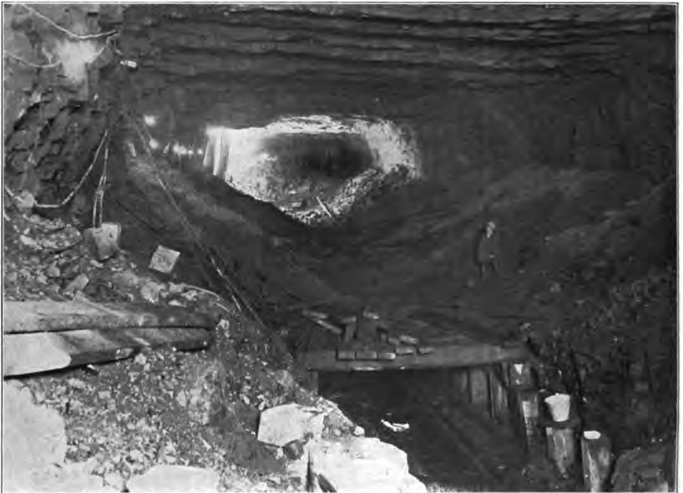
Fig. 6—Break-up Showing Heading and Jumbo Timbers.
