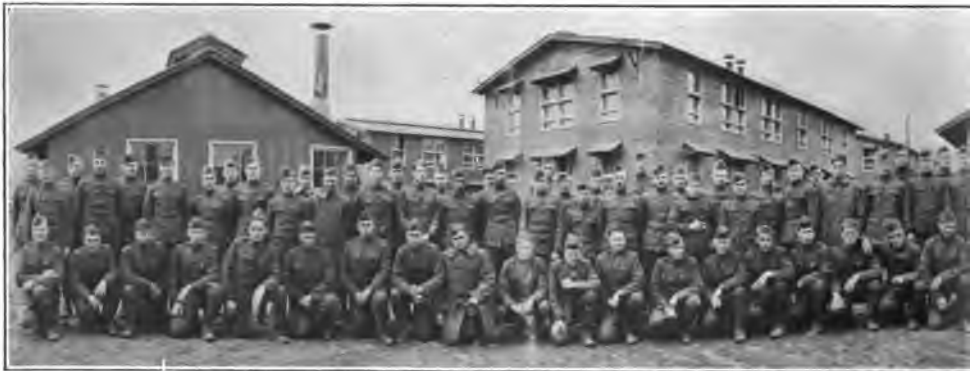
PART OF BATTERY "F" This detachment was detained in France
