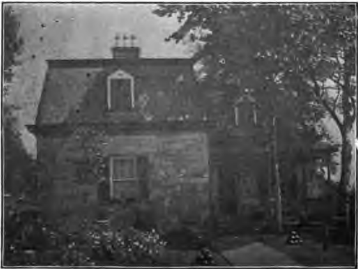
The Superintendent's Lodge at the National Cemetery, constructed of the stone taken from the famous "stone wall." (See page 191)
