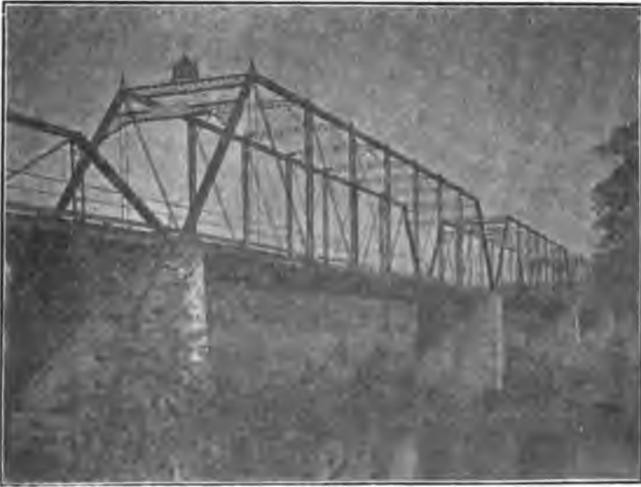
The Free Bridge over the Rappahannock River to Stafford Heights. (See page 171)
